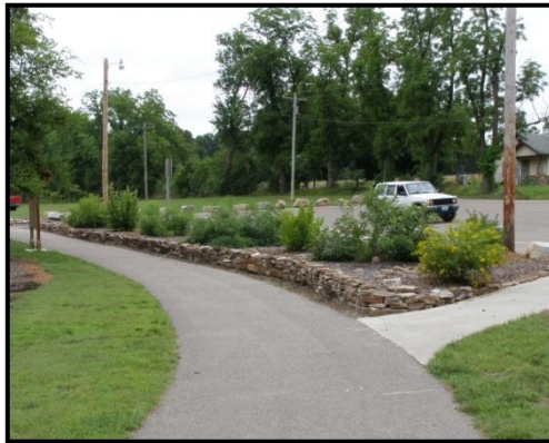
Parking Lot Bio-Retention Cell
