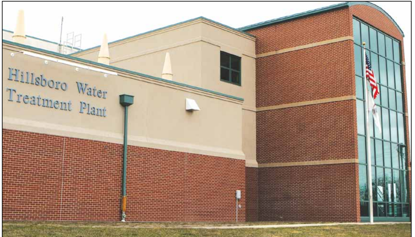
During a special meeting on Tuesday, March 6, the Hillsboro City Council hired Woodward & Curran, a water system management service from St. Charles, MO, to run the Hillsboro water department and treatment plant. Journal-News photo
