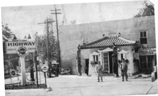
Gas Station South Side of FB Building
