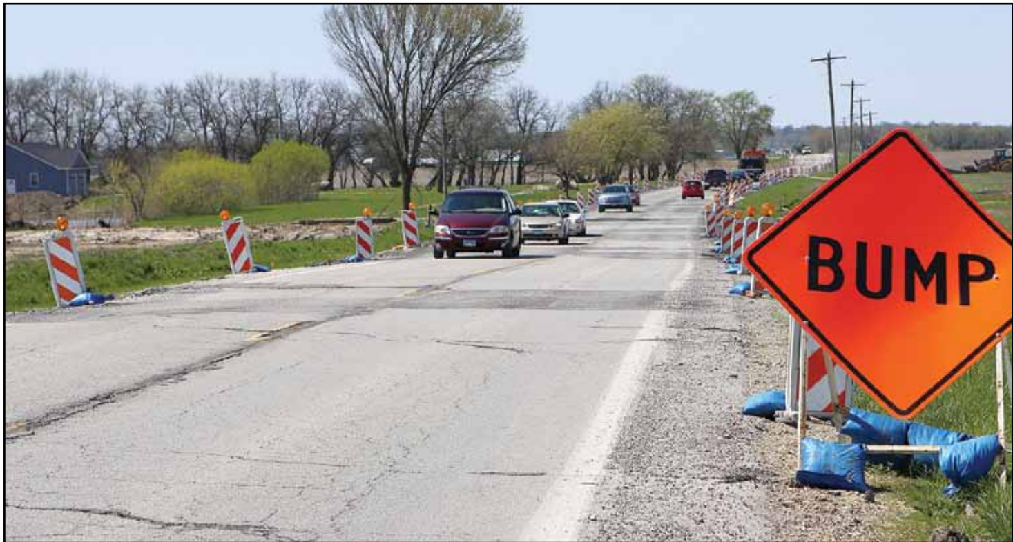
In February, the coal mine began longwall mining underneath Illinois Route 185, and subsidence from the mining has caused major damage to the road. Workers monitor the roadway 24 hours a day to make sure it's passable, and once the mining is finished, the coal mine will pay to have the road fixed under the guidance of the Illinois Department of Transportation.
