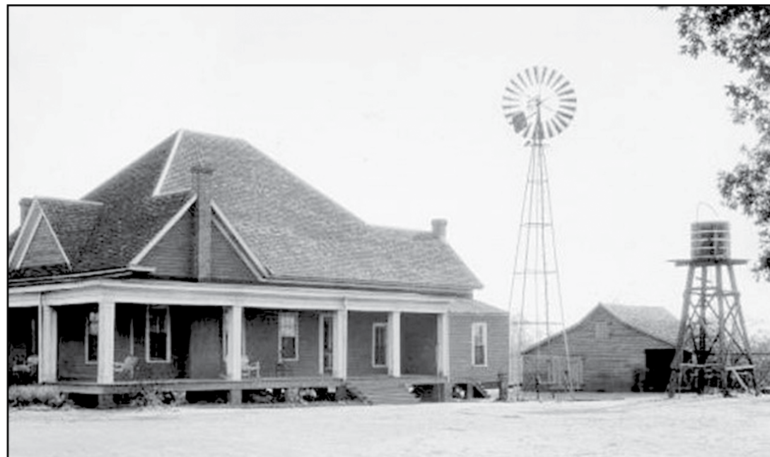
John McDaniel and his son, George, opened New Era Windmill Factory in Litchfield in 1892, going on to display their windmill in the 1904 World's Fair. The photo above shows the New Era Wind Mill powering a pressurized, elevated water delivery system for domestic, indoor plumbing in an isolated, rural area in Alabama in 1927.
