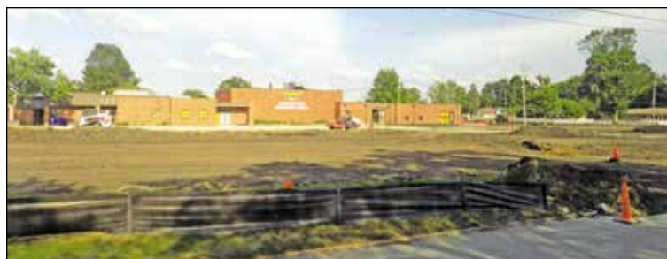
Parking lots dug up at Mid-Prairie East Elementary.
