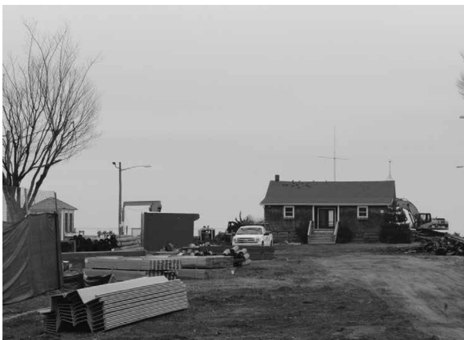
Work is progressing on the Bellport Marina Dock. Officials say it's still on target for an April 1 completion.
