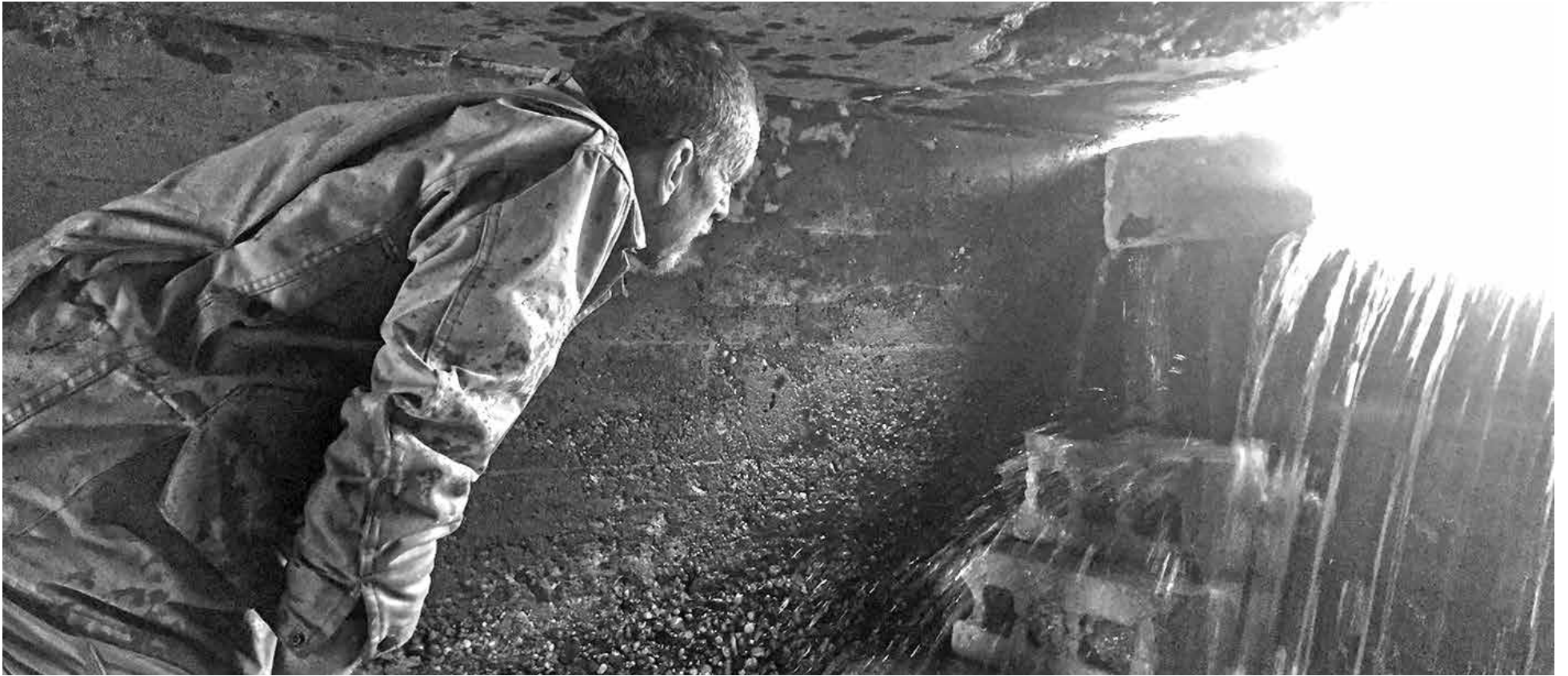
Seatuck wildlife biologist Mike Bottini looks at the concrete staircase created for otters to travel over the dam at Little Seaturk Creek and under East Moriches Boulevard in Eastport.
