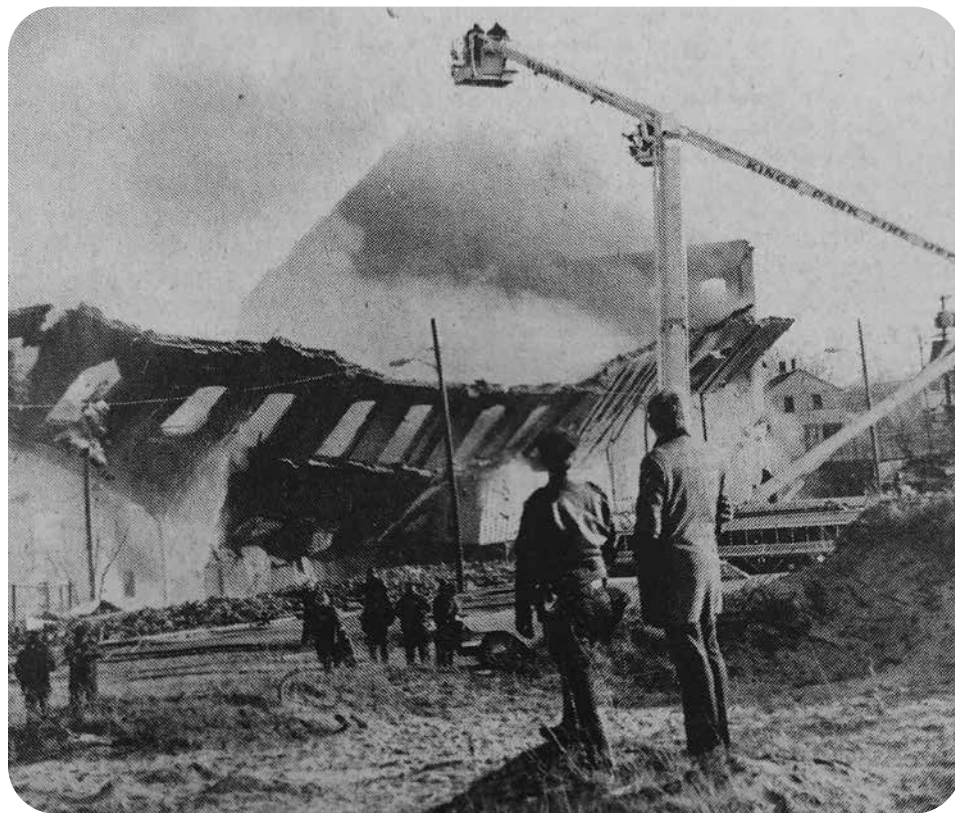
Wall comes down and snorkel pours water onto debris in an attempt to dampen the flames and smoke emerging from the fire that engulfed the complex. Fire started on second floor and was brought under control by about 5 p.m.
