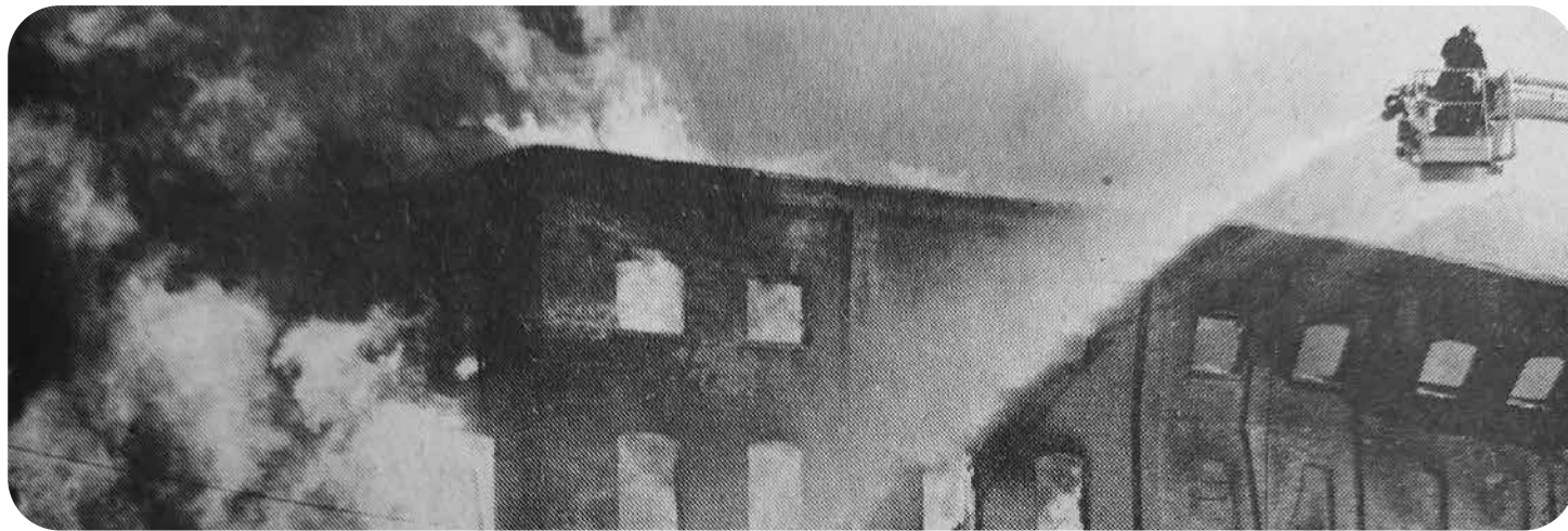
Flames pour out and wall starts to collapse as volunteer firefighters tackle fire Monday that destroyed about one-third of the old Lace Mill, now Island Industrial Park, on West Main Street in Patchogue. The wall seen faces west and was brought down as a safety factor.
