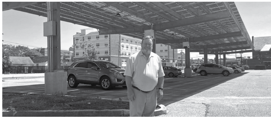
Village of Patchogue BID executive director Dennis Smith stands in front of the newly installed and functioning solar carport behind the Patchogue Theatre for the Performing Arts.
