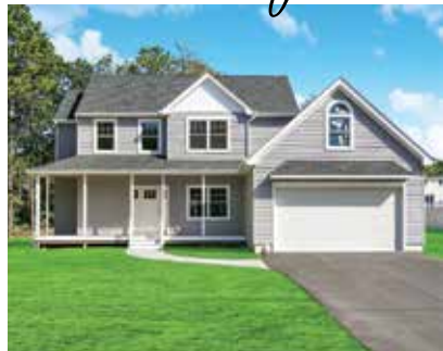
Bellport - New Construction
