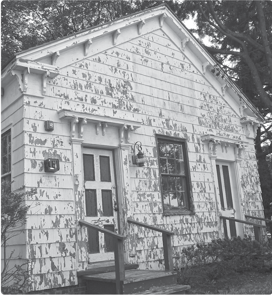
Renovations are underway at the Swan River Schoolhouse in East Patchogue.
