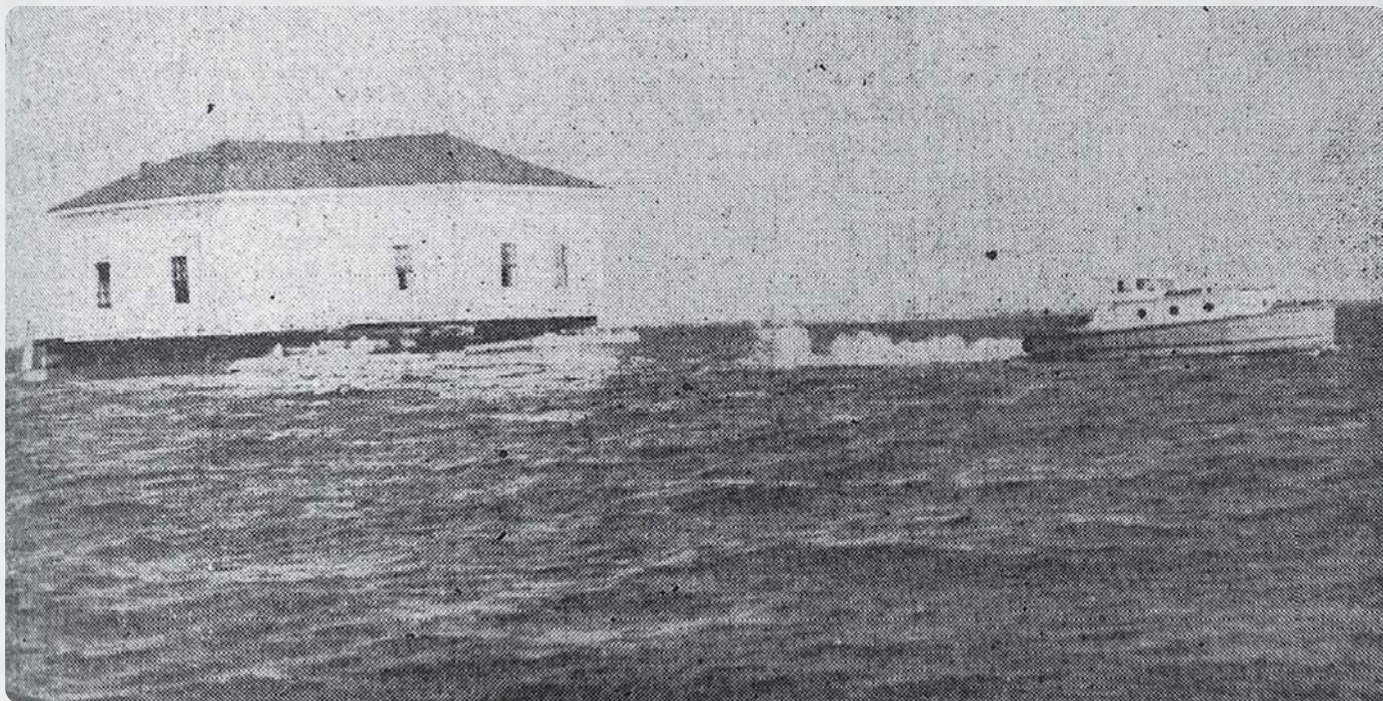
From the Sept. 30, 1948 edition: One of the buildings formerly used at the Forge River Coast Guard station was recently towed to a new site in Blue Point. The building was purchased and moved by the Davis Brothers Engineering Company, and is now located on the company's property on Barteau Avenue, Blue Point. It will be used as a garage-workshop. The main building at the Forge River station was floated to Ocean Bay Park, Fire Island, Saturday, where it will be partitioned and made into 10 double and single rooms for vacationers at the beach.
