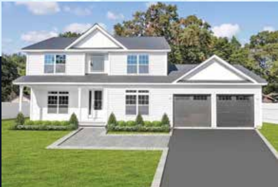
New Construction 185 SOUTHAVEN, MEDFORD
