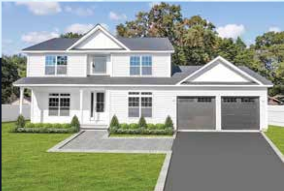
New Construction 185 SOUTHAVEN, MEDFORD
