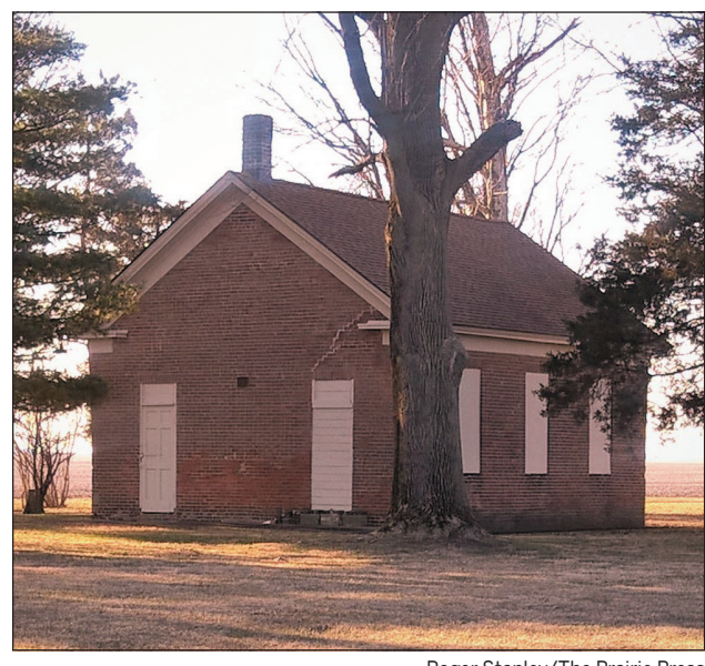
Roger Stanley/The Prairie Press Pine Grove School is the oldest surviving school building in Edgar County. It was built in 1867.
