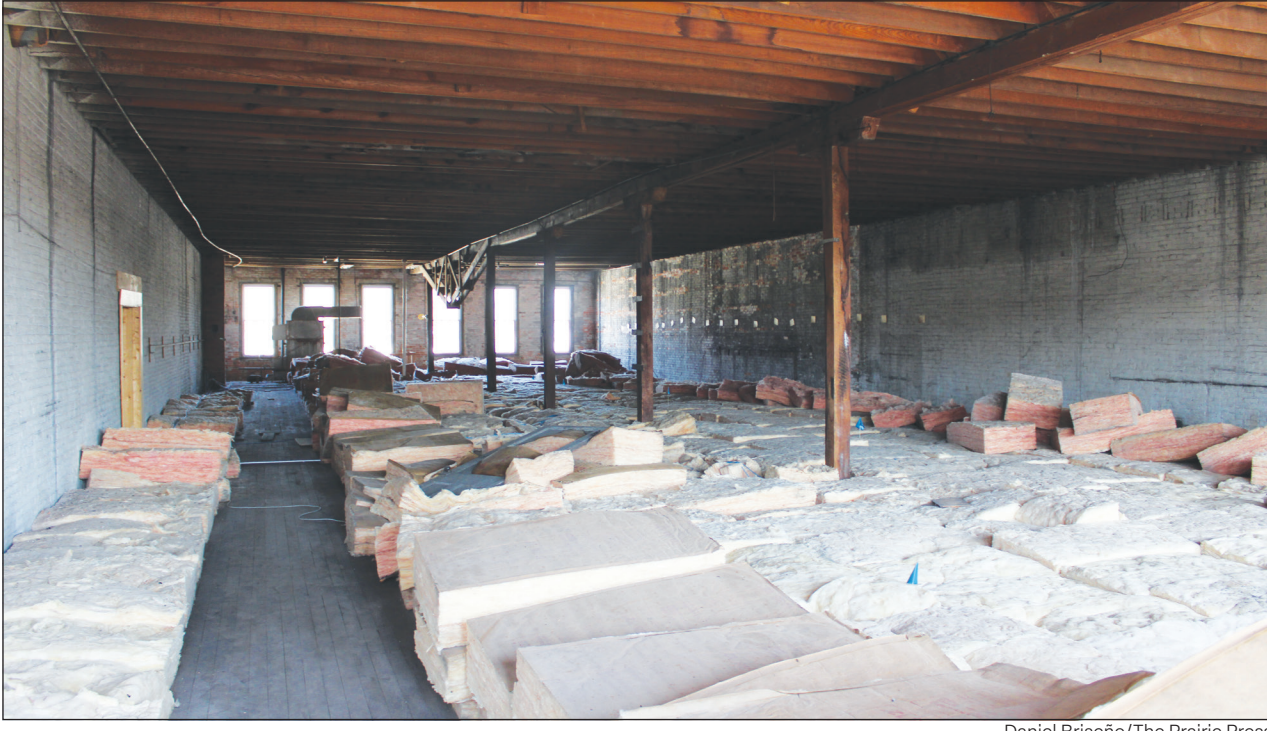
The Marshall Public Library first applied for a $2.5 million dollar grant to renovate a 3,000 square-foot section on the library's second floor. The first application was denied.
