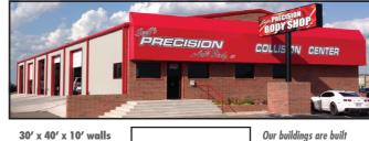
30' x 40' x 10' walls 4" 3500 lb Floor w/ Fiber mesh 24" Pier holes w/rebar 26 Ga. Color R-Panel 40 yr.
