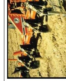
Fig. 12. Moderately dry topsoil is being replaced on the affected site now that Phase 1 deep ripping of the compressed subsoil is complete.
