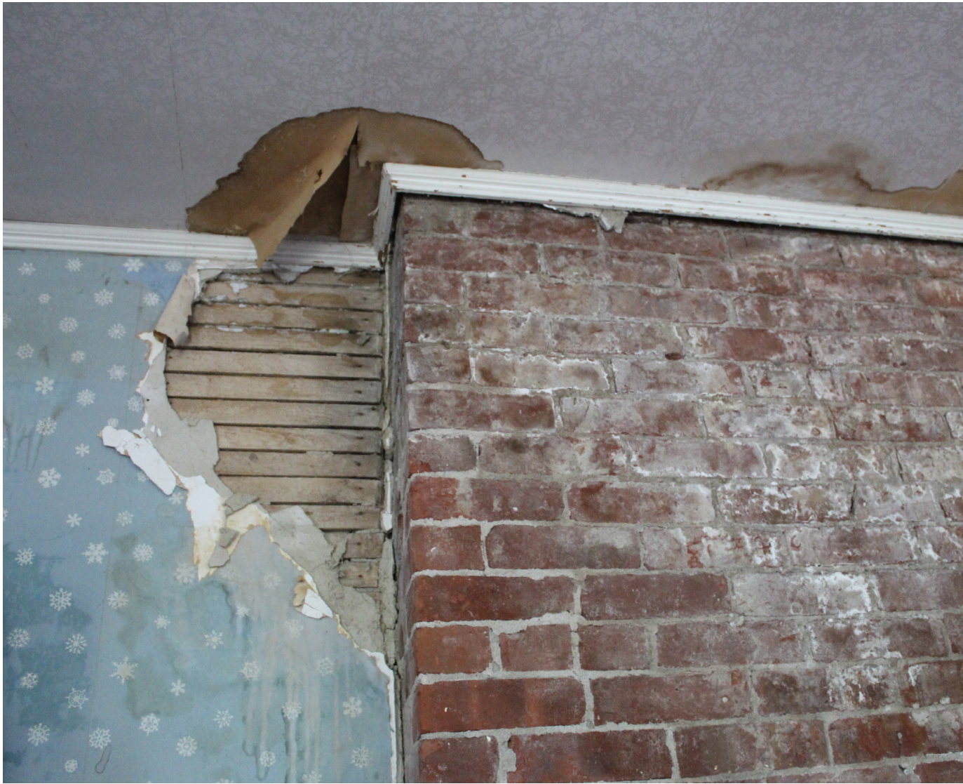
A closeup of damage around a chimney. We assume it was a leak. The flashing got fixed but this mess needs to be repaired.
