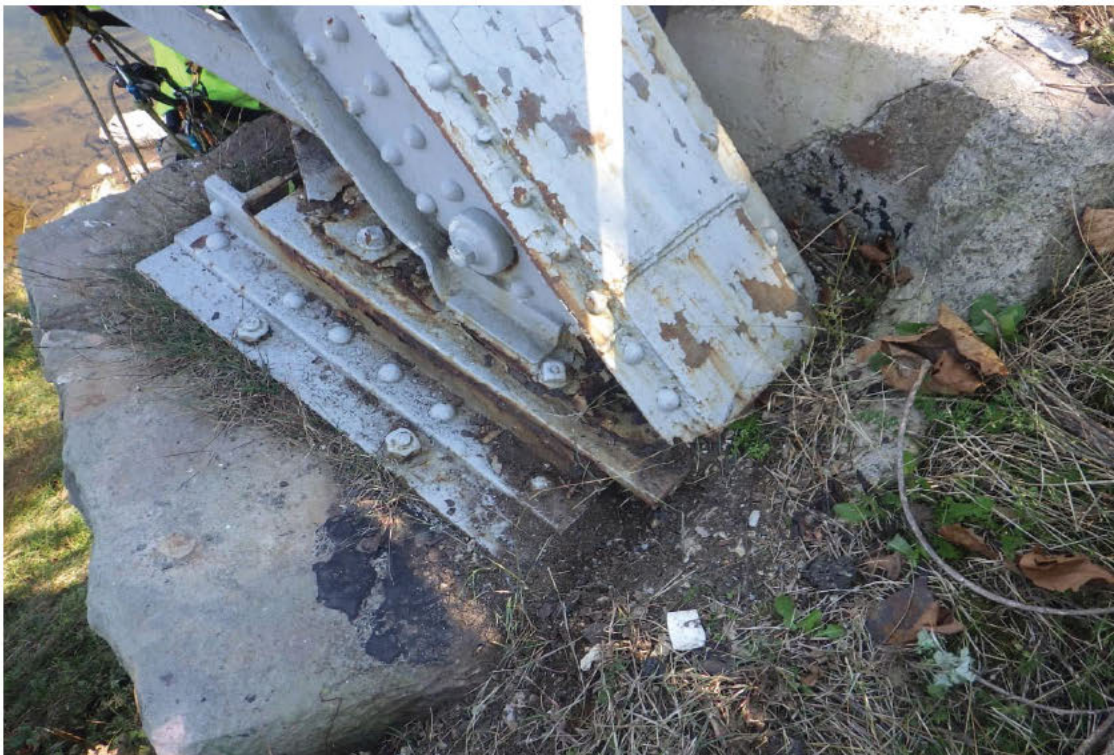
72. General view of the Left Truss Bearing at the Near Abutment.
