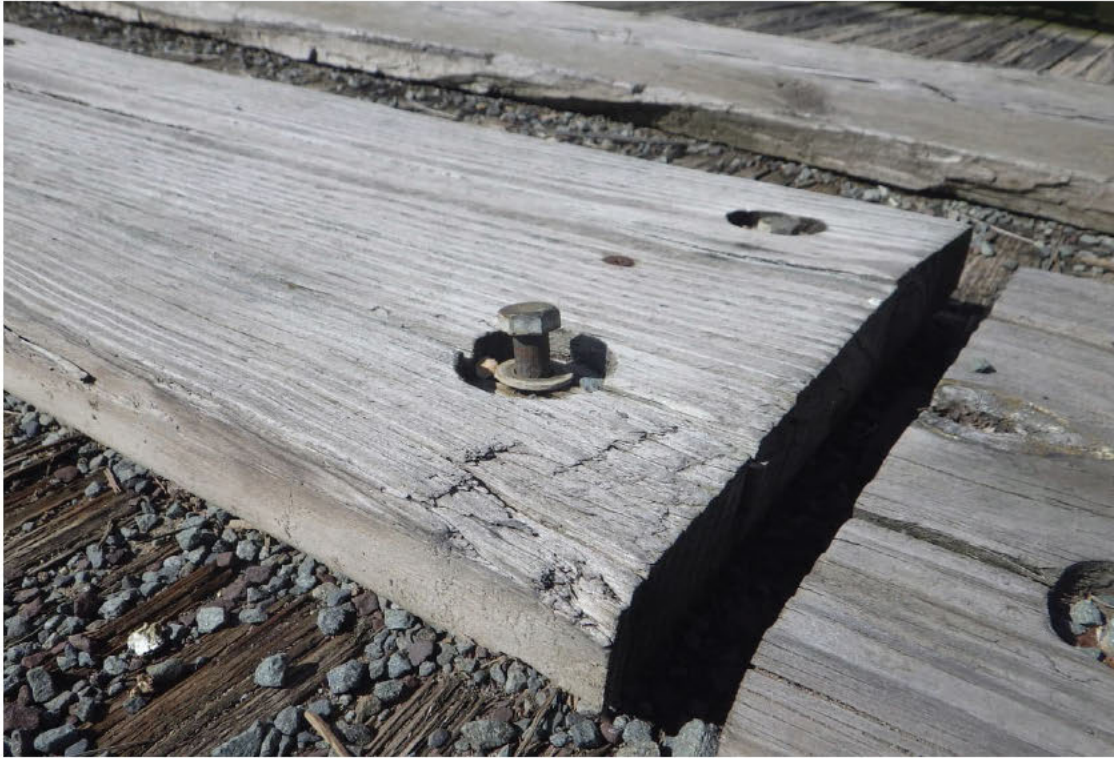
13. Typical loose fasteners protruding from the running planks.
