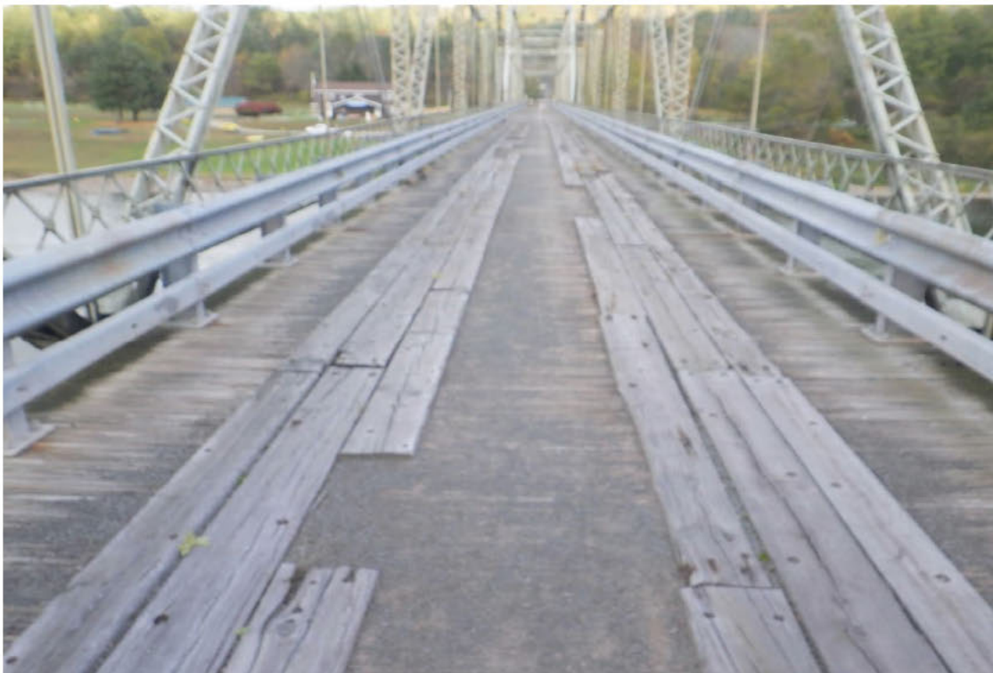
10. Top of deck in Span 1, looking ahead.
