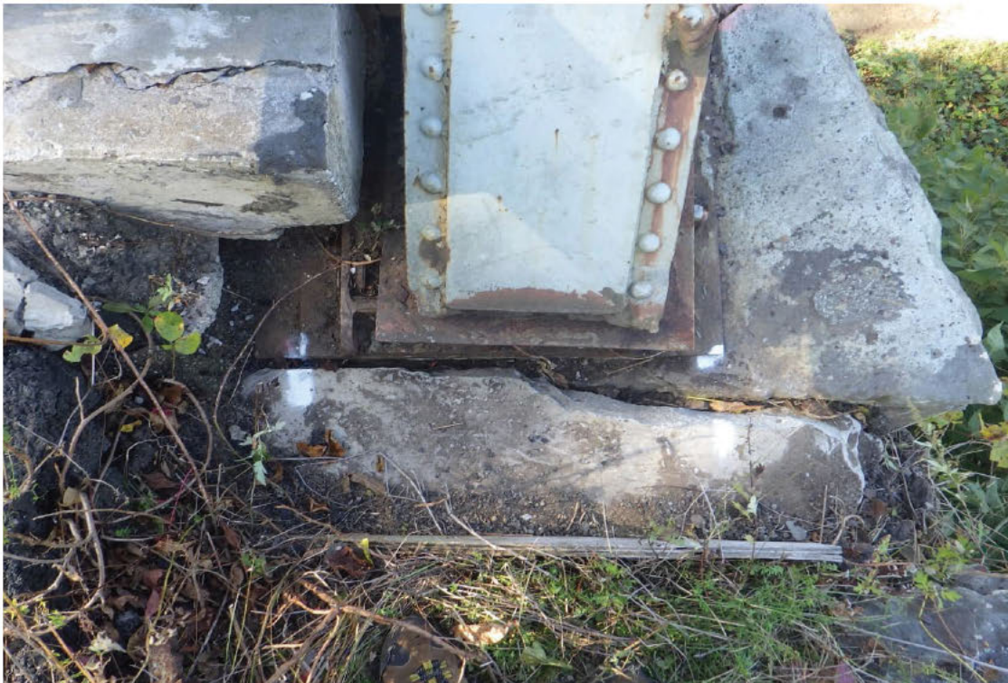
114. Repair adjacent to the left truss bearing at the Far Abutment.
