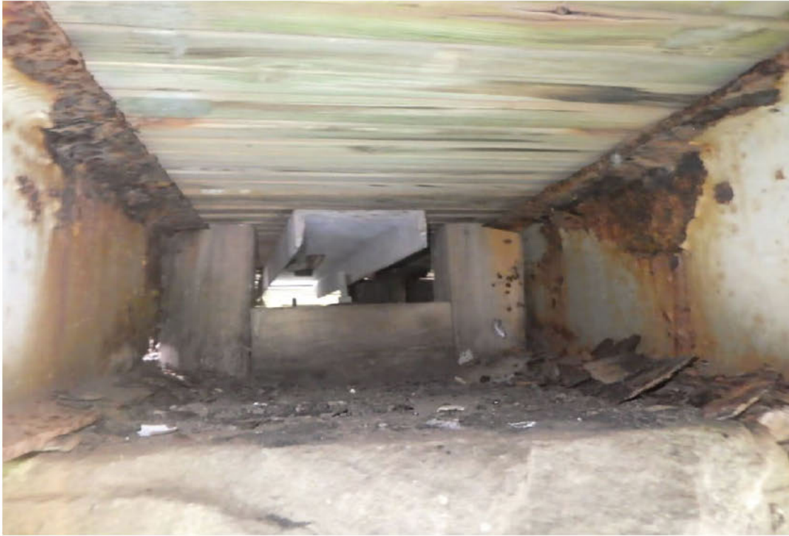
57. Timber cribbing in Bay 10 over Pier 1, looking back.
