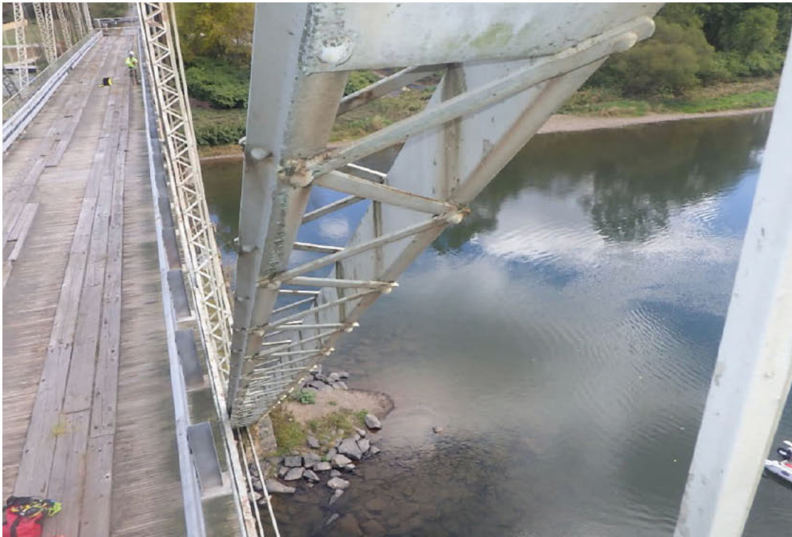
22. Typical diagonal condition, M9-L10, Right Truss in Span 1, looking ahead.
