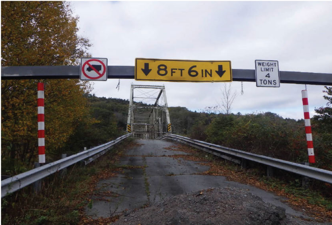
7. PVC tubes detached and hanging from far clearance bar.
