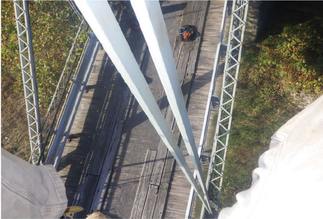
23. Typical vertical condition, L2-U2, Left Truss in Span 1.
