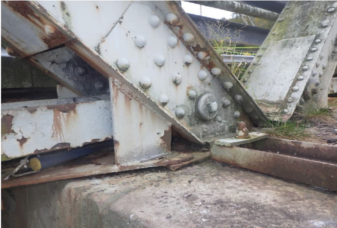
77. Left truss bearings at Pier 1, looking right.
