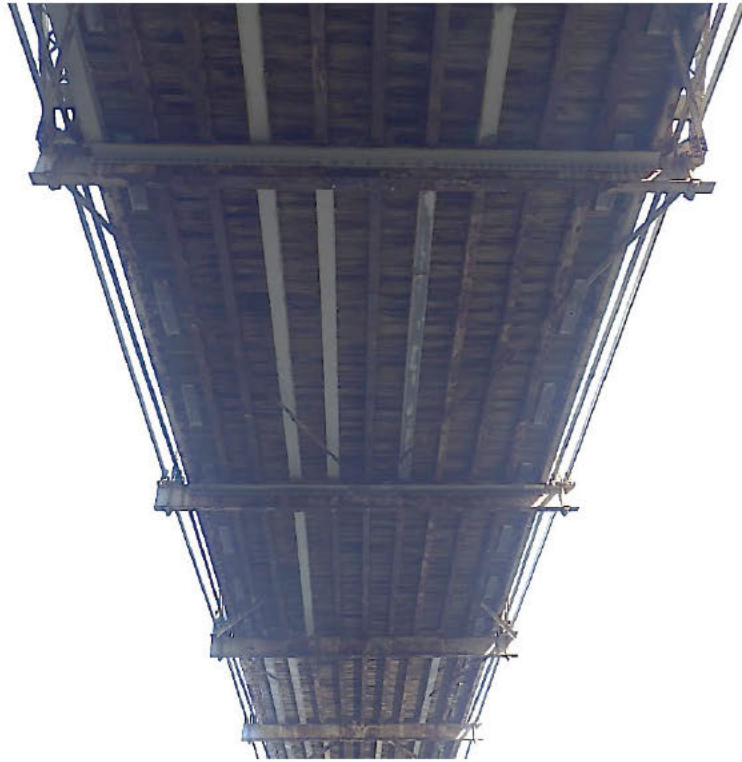
19. General underside of Span 1, looking ahead.
