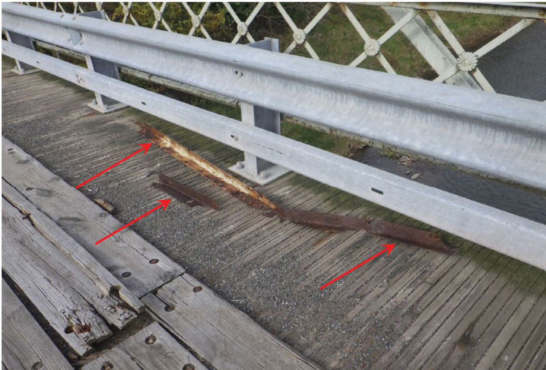
70. Removed left lower lateral brace, Bay 4 in Span 1. (Removed during inspection)
