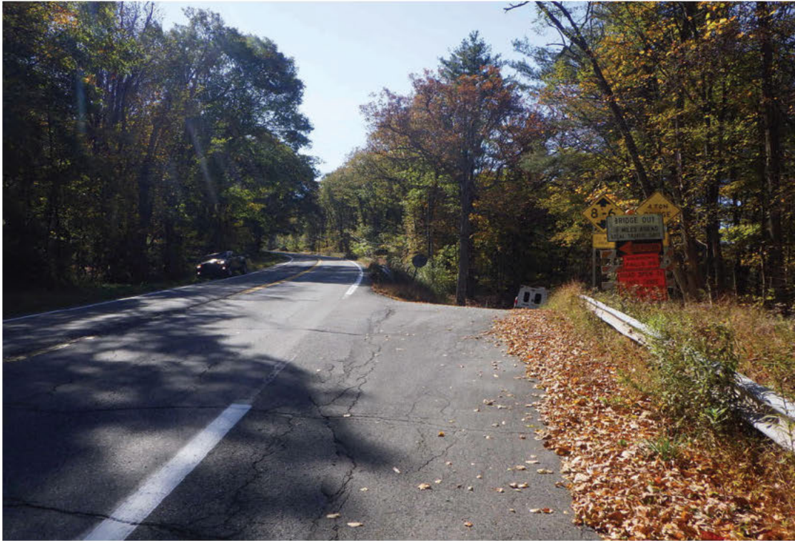
129. Far approach sign, looking south on Route 97 at North Skinners Falls Road intersection.
