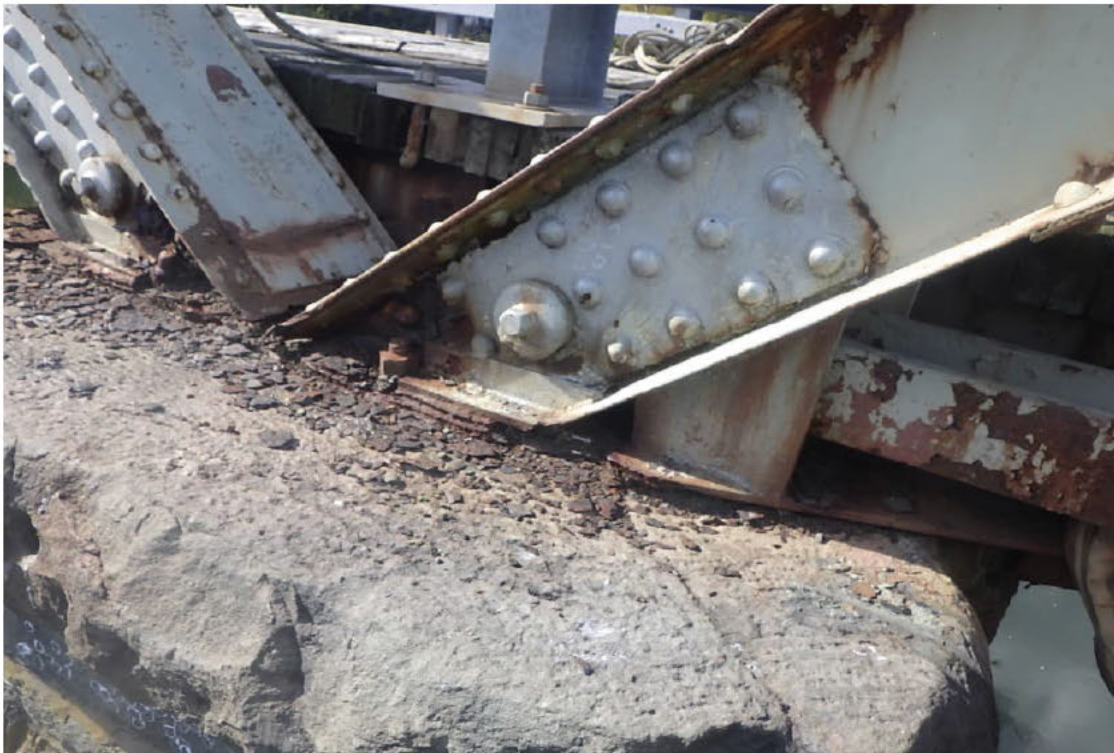
78. Right truss bearings at Pier 1, looking left.
