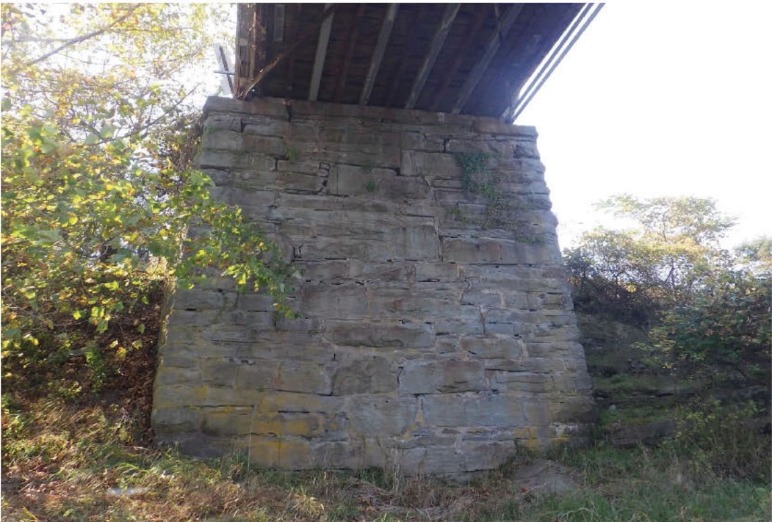
86. General view of the Near Abutment.
