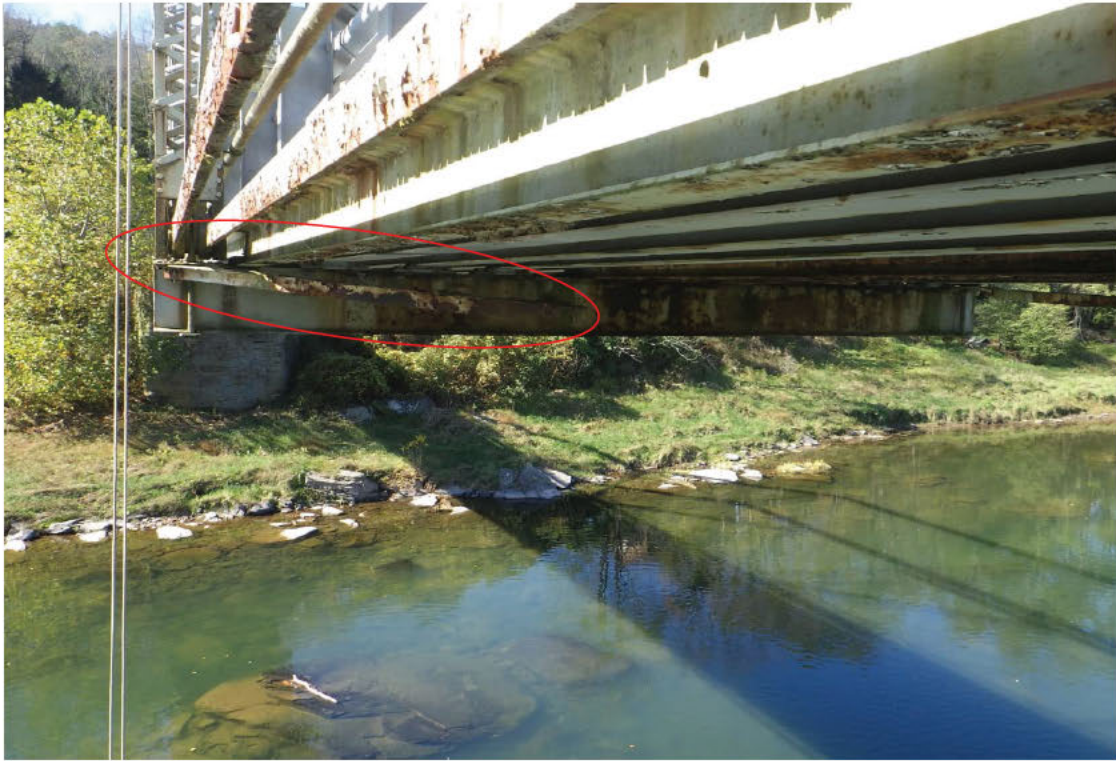
19. Partial length lower lateral bracing, Span 1 between FB 8 & 9. looking back.
