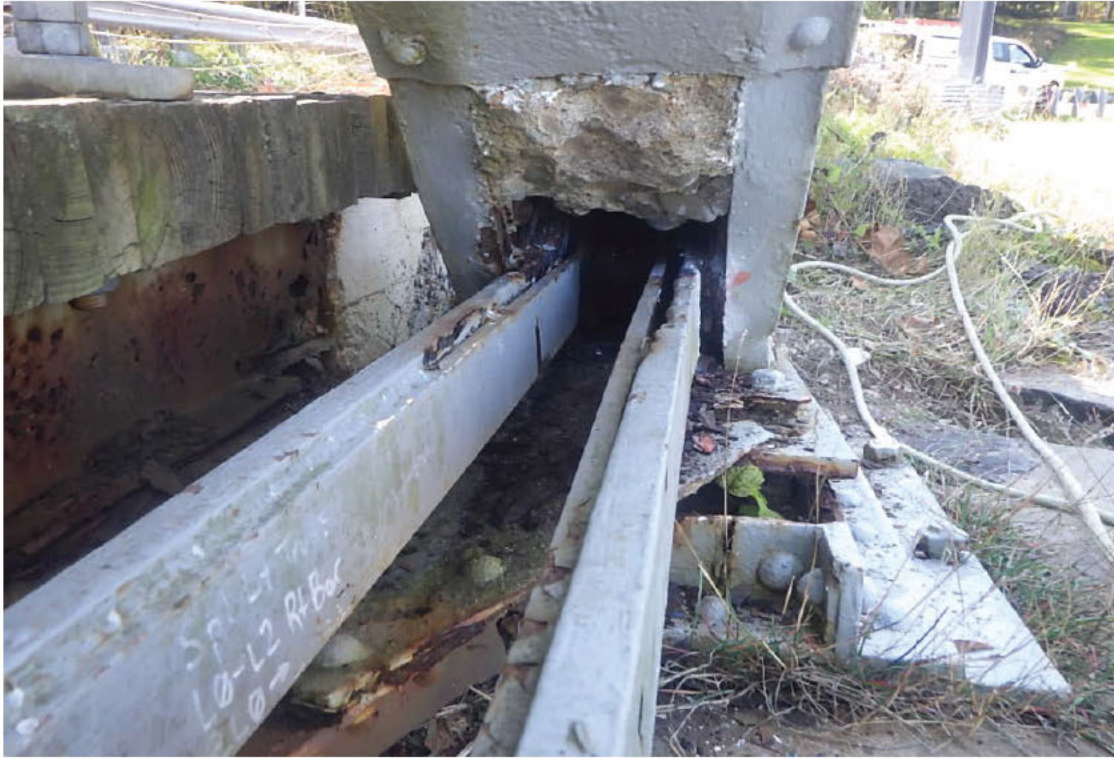
29. Bottom chord repair, L0-L1 at L0, Left Truss in Span 1.
