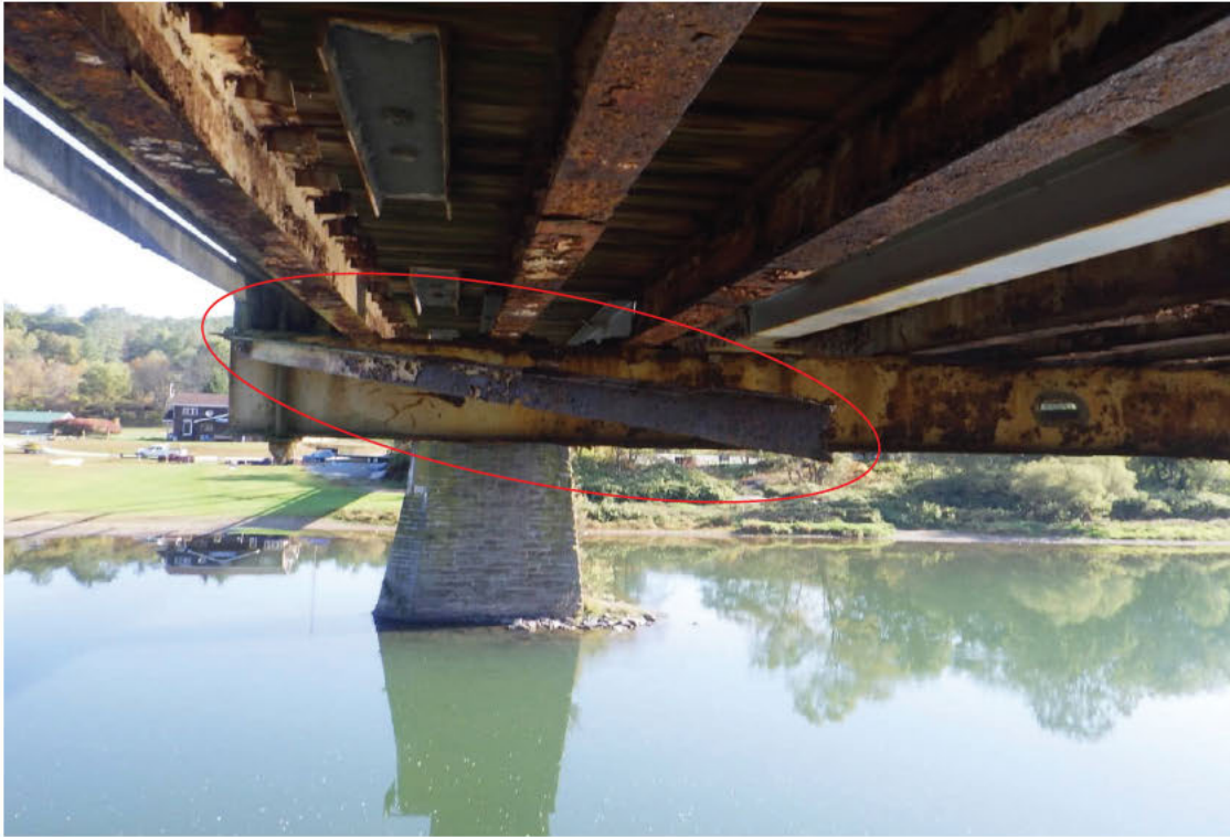
71. Remaining cantilevered section of left lower lateral brace, Bay 4 Span 1.
