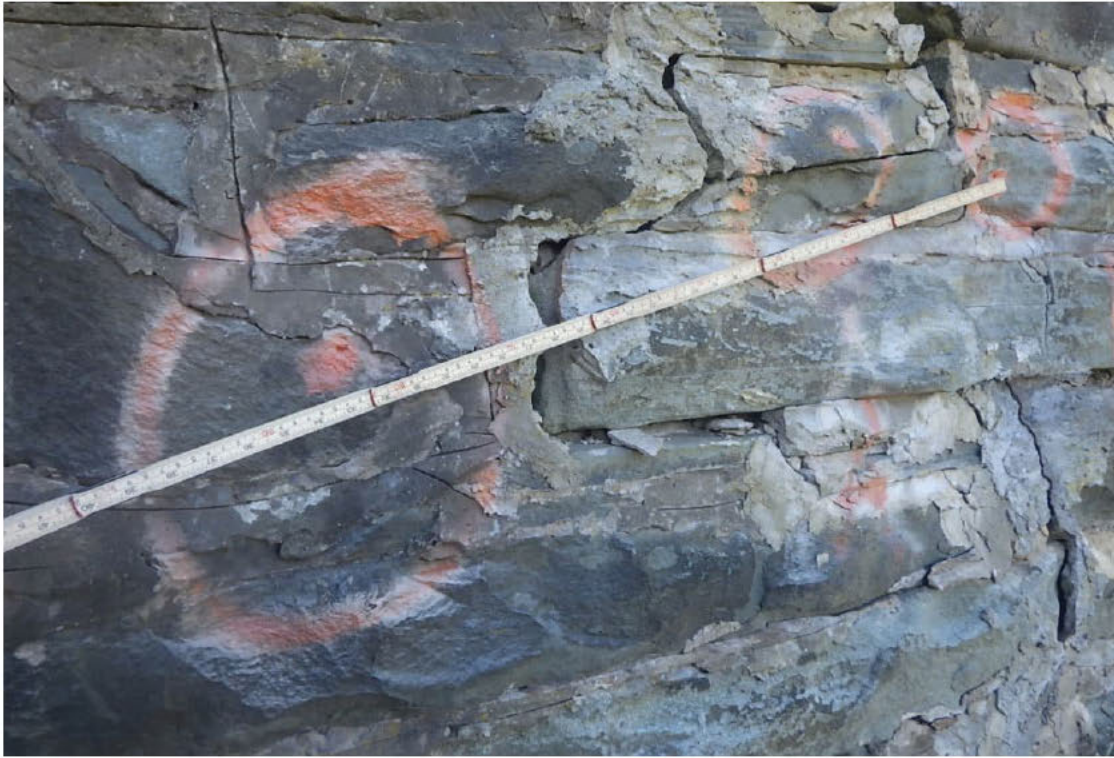
121. Monitoring point A' to B at the Far Left wingwall.
