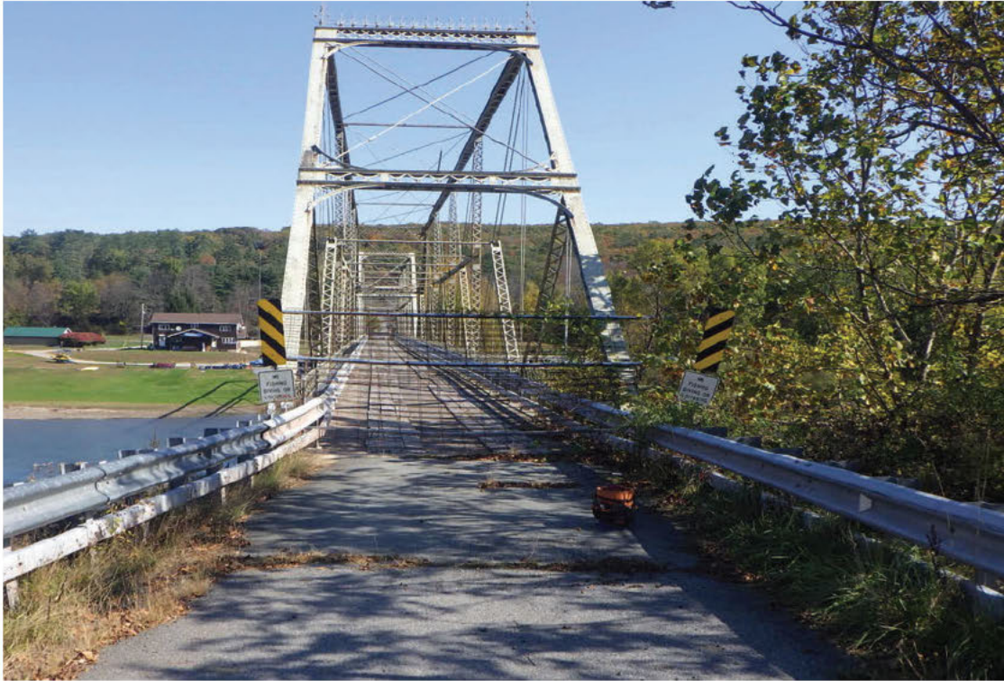
5. Near portal with reinforcement mesh used to restrict access to bridge.
