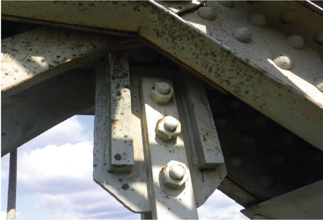
37. Retrofit vertical, L10-U10, Left Truss, Span 2.
