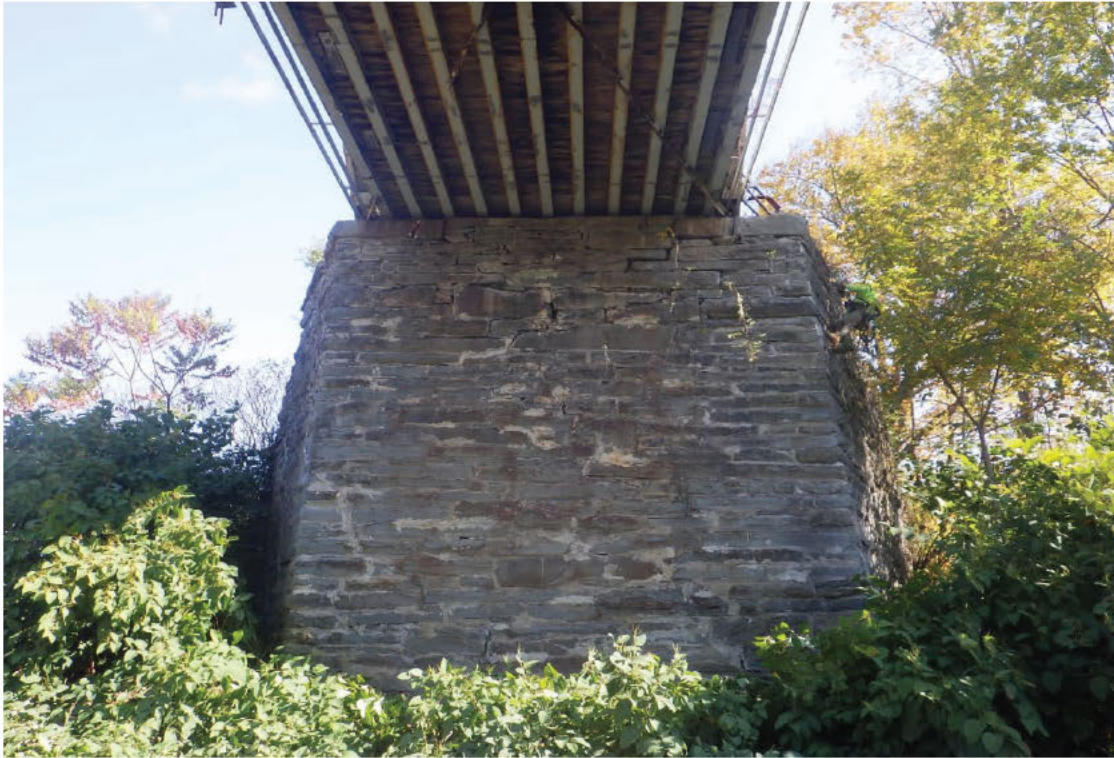
109. General view of the Far Abutment.
