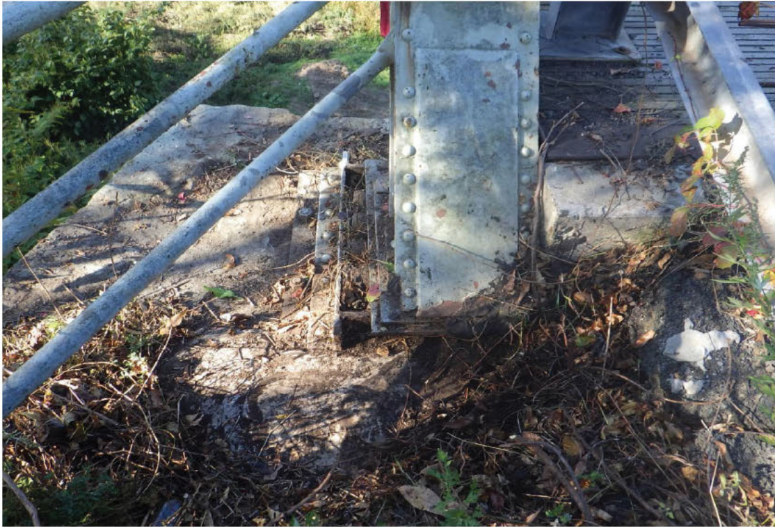
83. General view of the Right Truss bearing at the Far Abutment.
