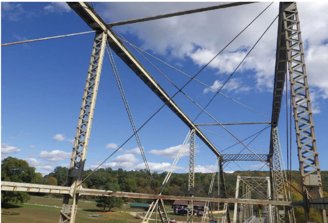
42. Typical sway bracing, M6-U6 in Span 1.
