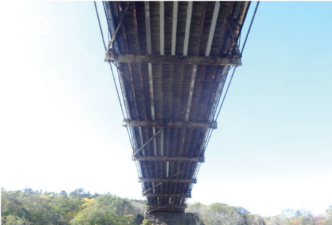
20. General underside of Span 2, looking back.
