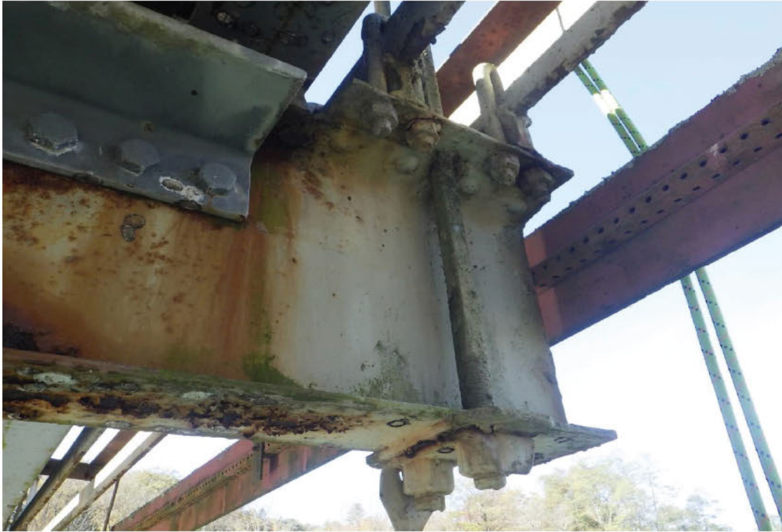
47. Typical floorbeam connection, FB9, Left Truss in Span 1, looking back.
