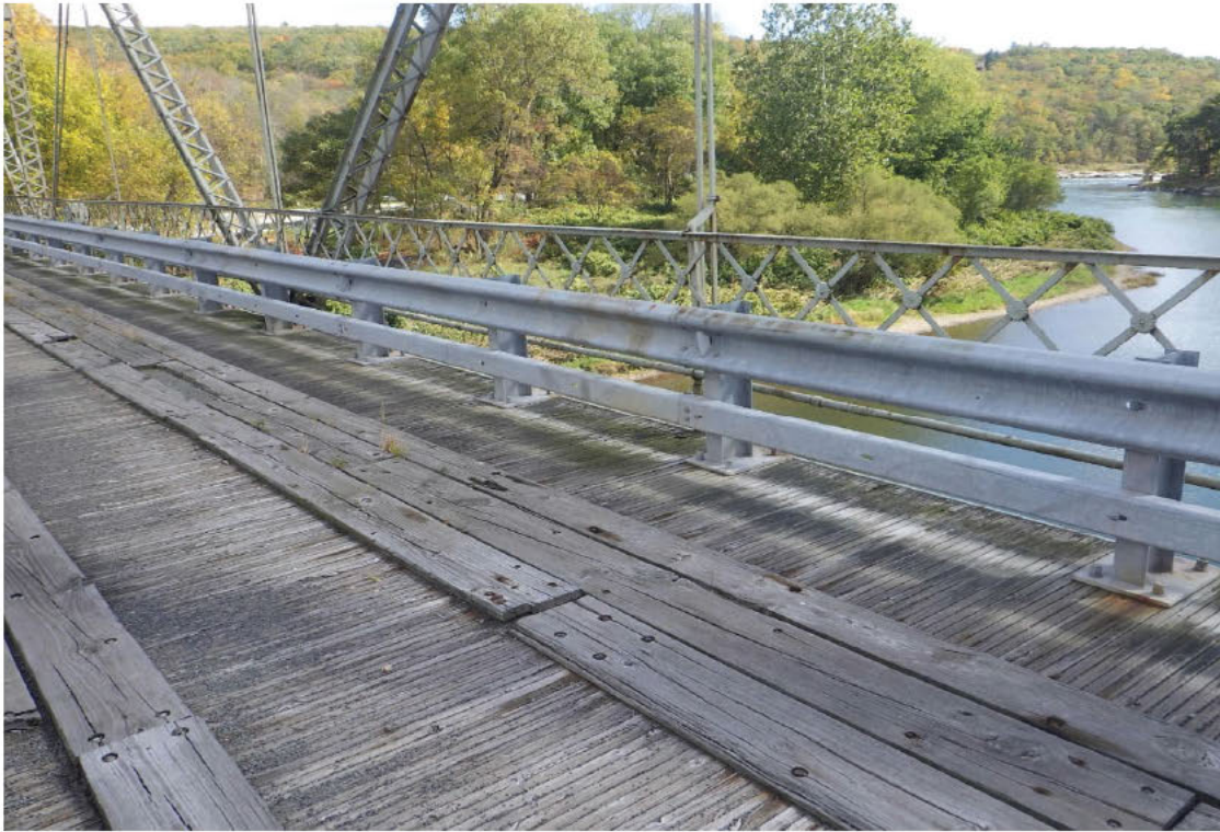
17. Typical bridge railing, looking right.
