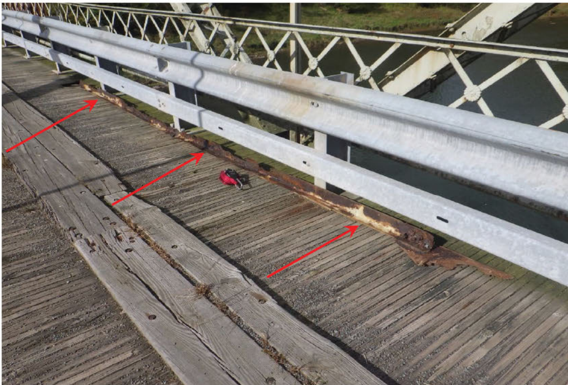
68. Removed right lower lateral brace, Bay 12 in Span 1.
