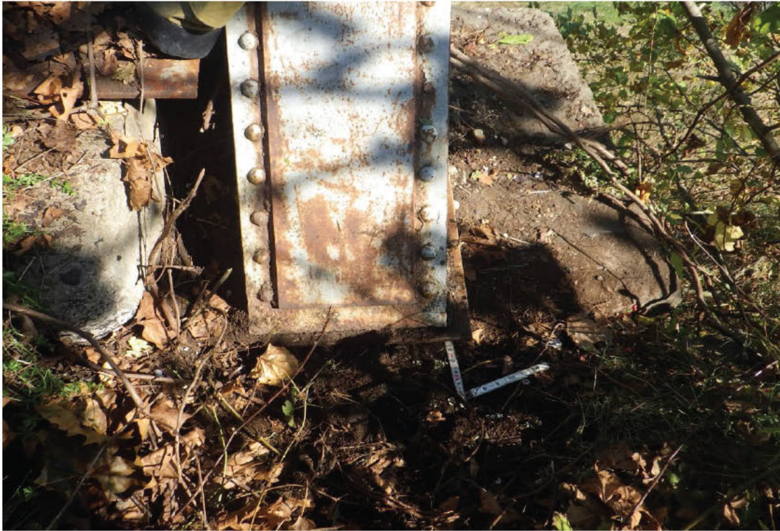
75. General view of the Right Truss bearing at the Near Abutment.
