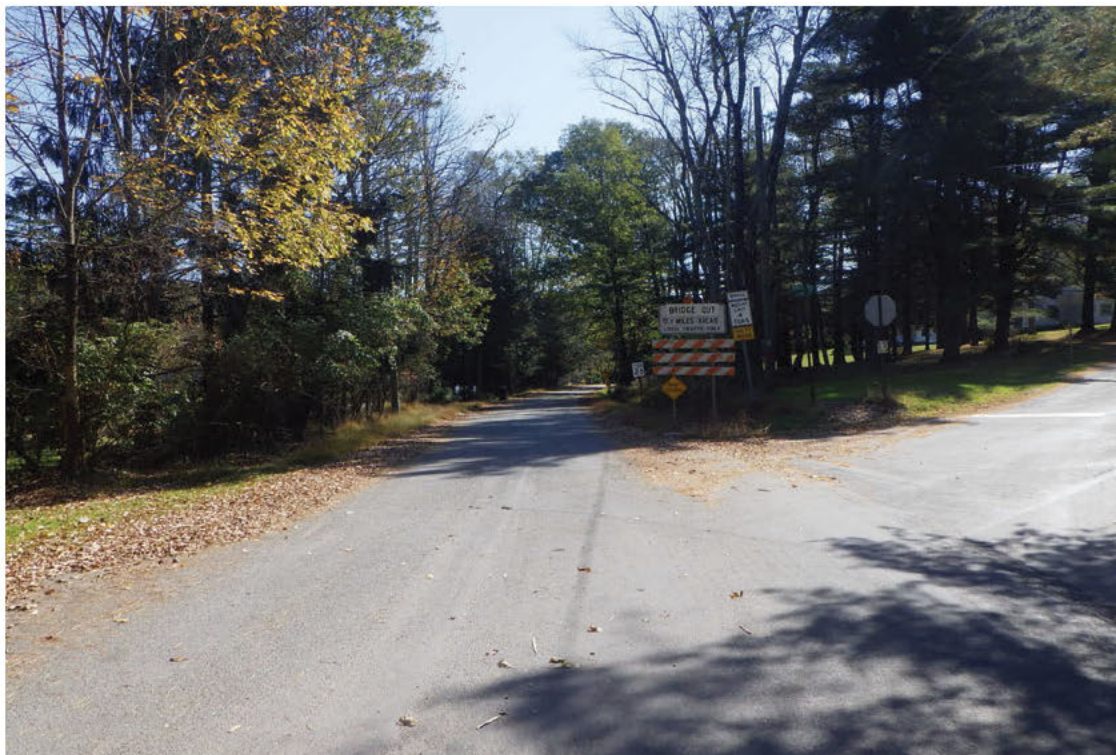
126. Near approach sign on Calkin Road near south River Road intersection.
