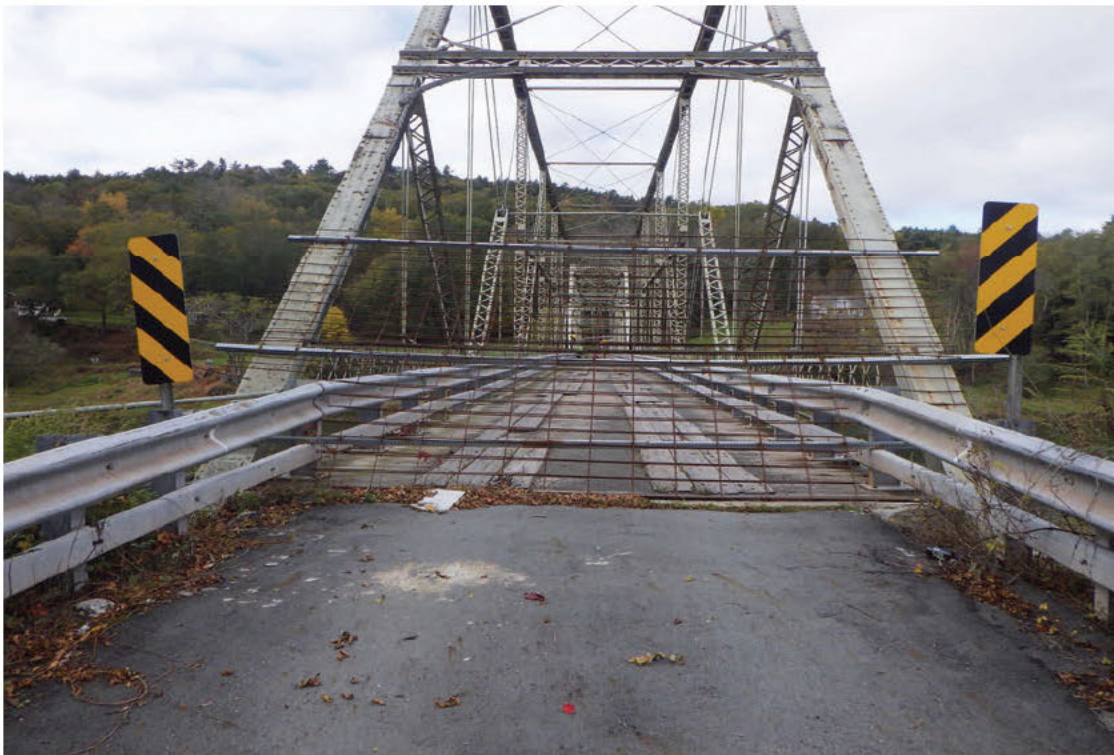
6. Far portal with reinforcement mesh used to restrict access to bridge.
