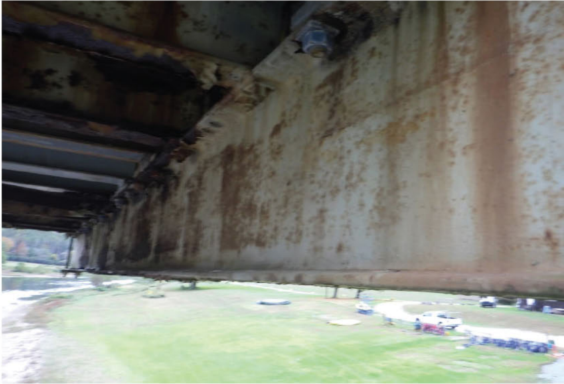
45. Typical view of Floorbeam 7 in Span 2, looking far left.
