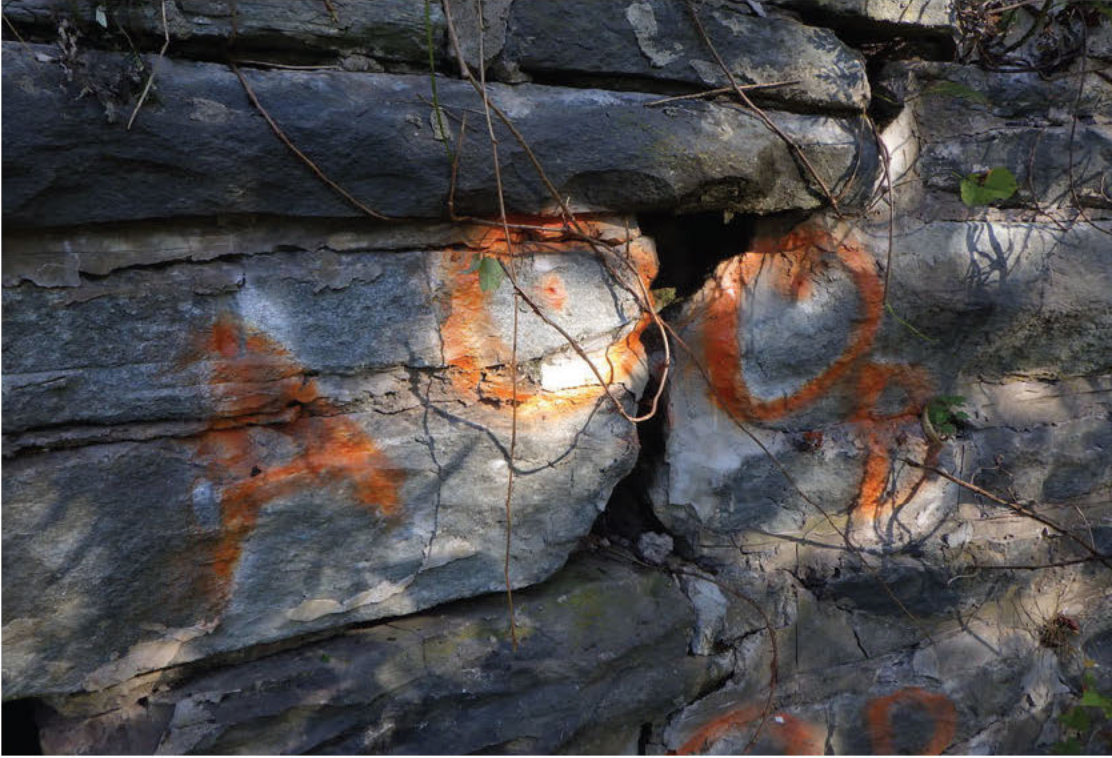
123. Far Right wingwall monitoring point A-B, no change from previous inspection.
