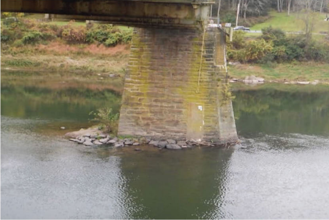
105. General view of the far face of Pier 1.
