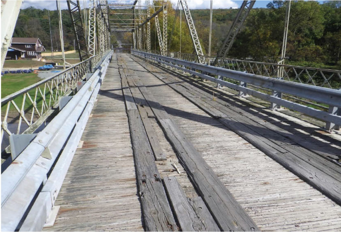
11. Top of deck in Span 2, looking ahead.
