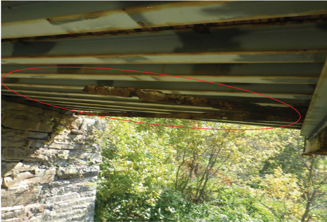
65. Left side Bay 12 Span 2
