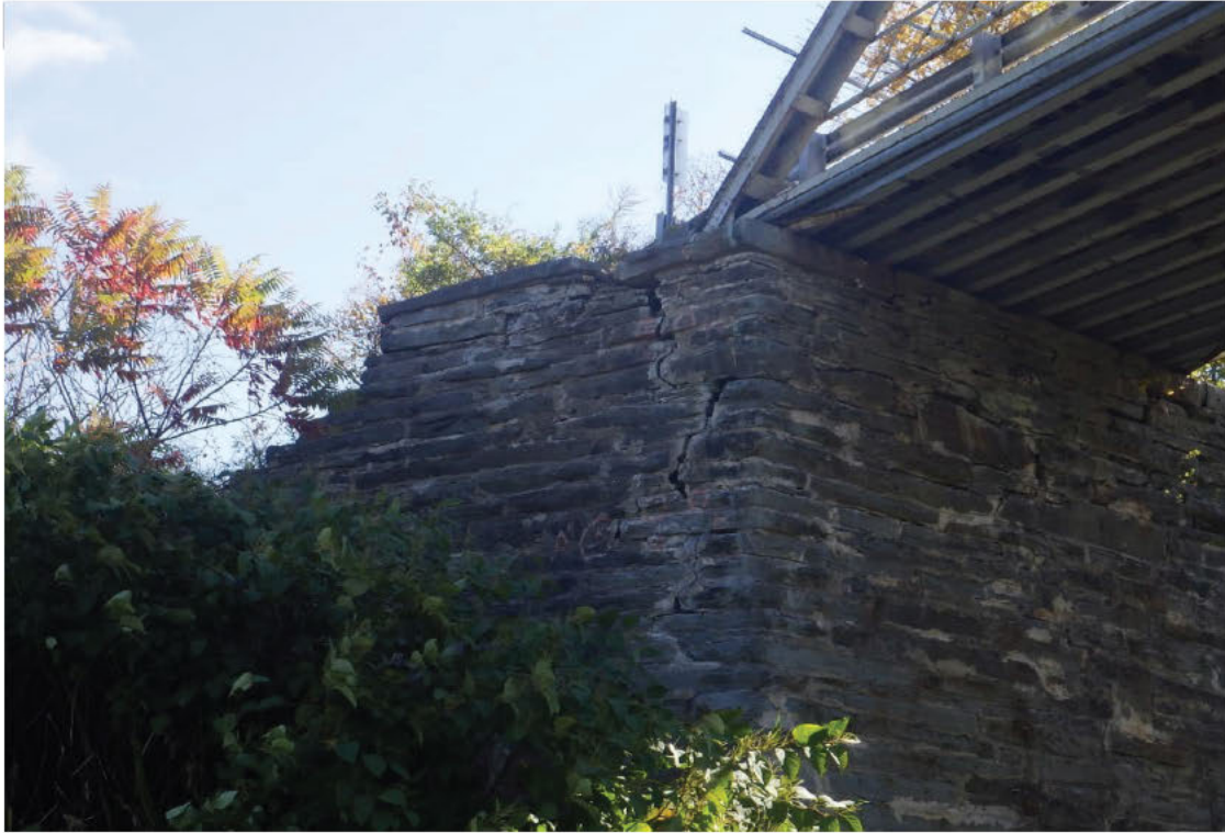
17. General view of the Far Left Wingwall.
