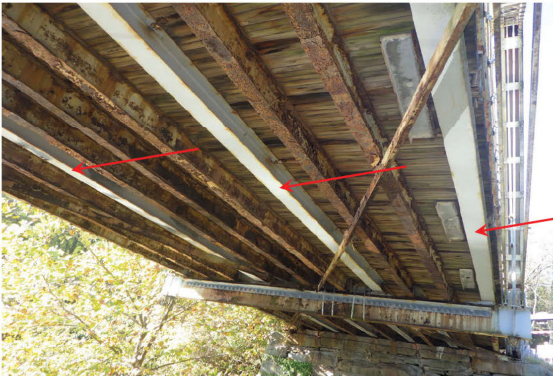
58. Typical newer stringer in Floorbeam Bay 2 of Span 1, looking back
