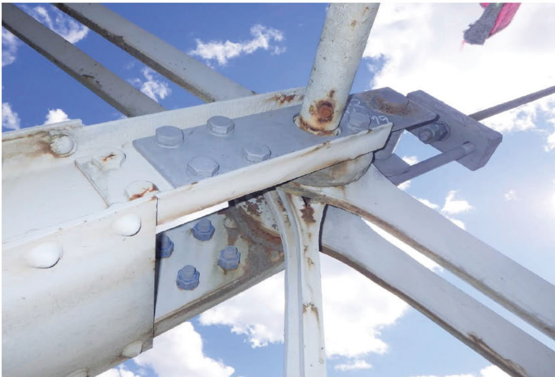
32. Retrofit U8-M9 at M9, Right Truss, Span 2.
