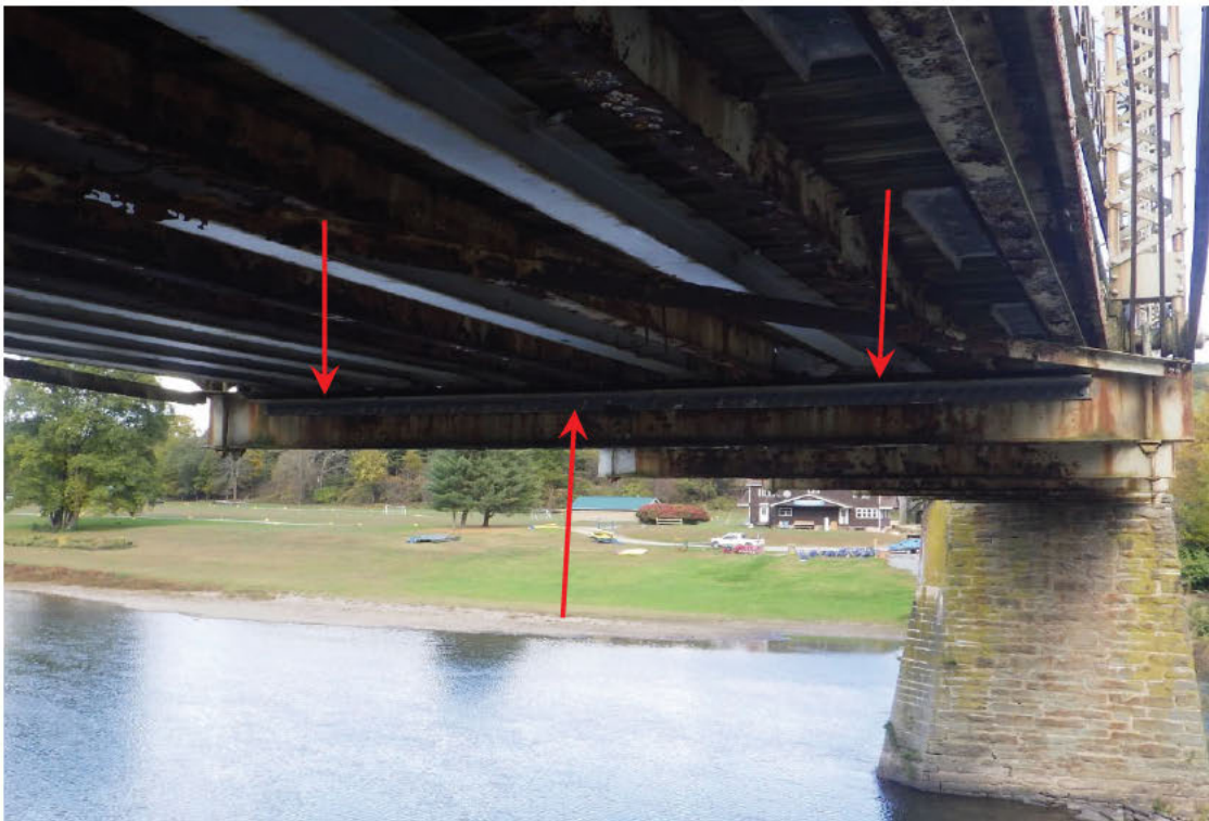
46. Angle repair to Floorbeam 8 in Span 1, looking ahead.
