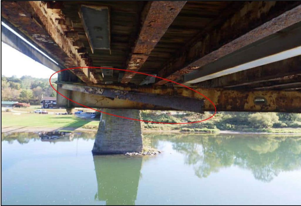
Photograph 7: Deteriorated cross bracing (October 2024).
