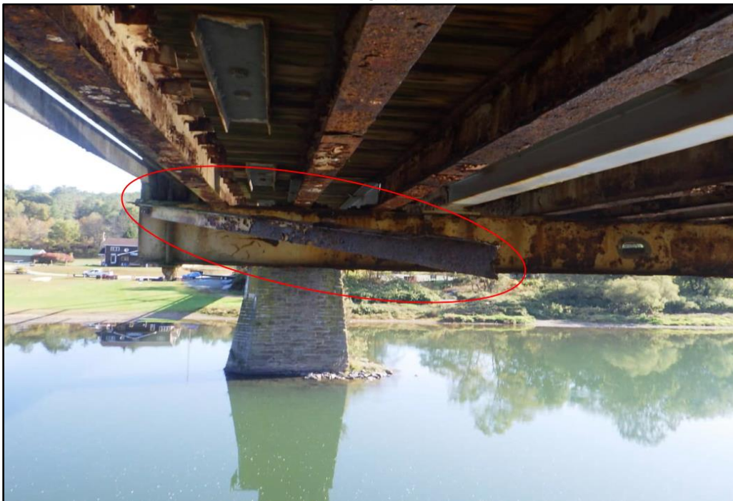
Photograph 7: Deteriorated cross bracing (October 2024).
