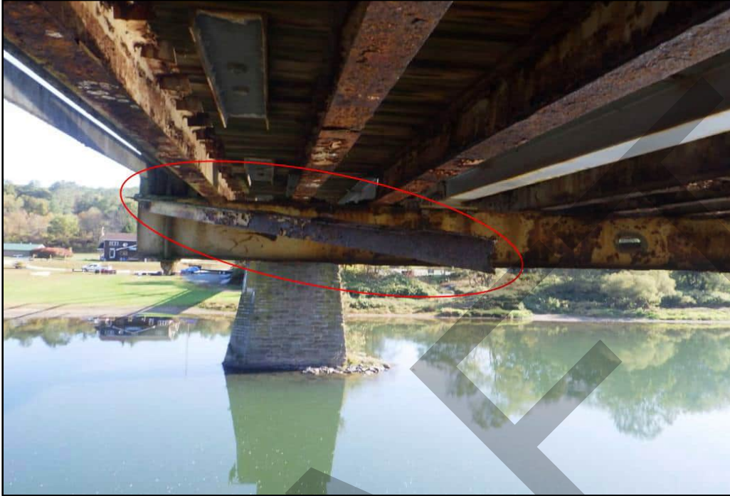
Photograph 7: Deteriorated cross bracing (October 2024).
