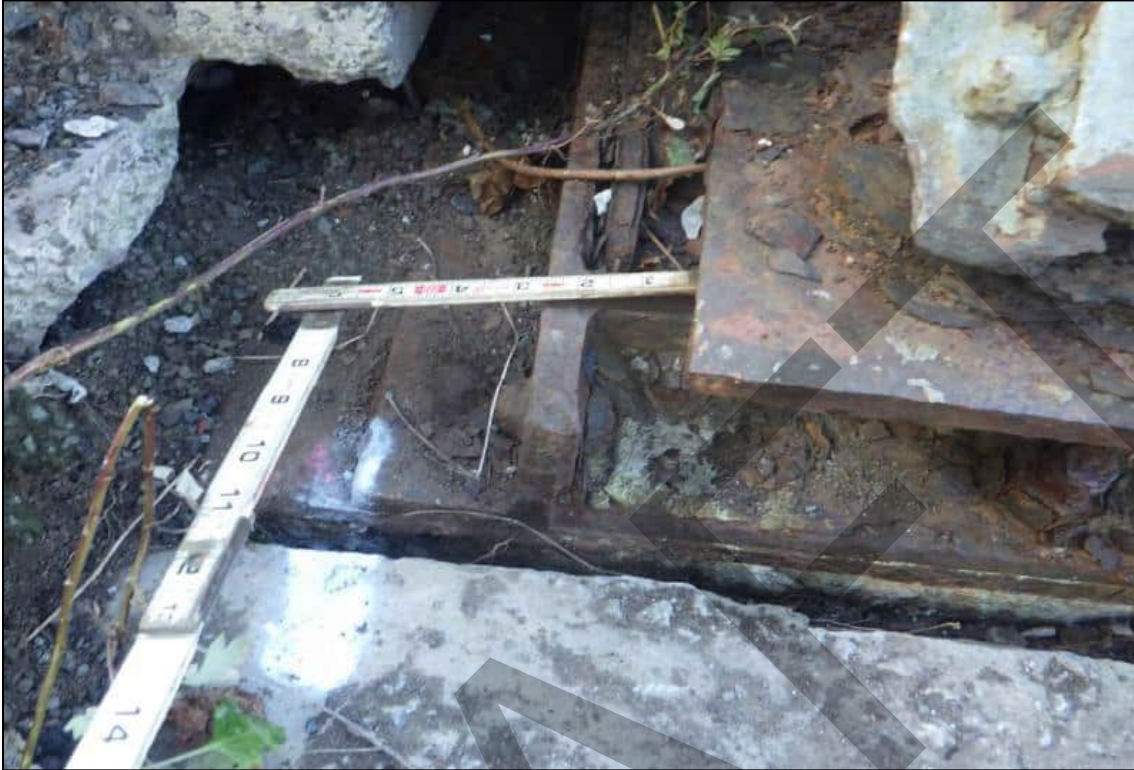
Photograph 5: Sole plate shifted left on the left truss bearing at the Far Abutment (October 2024).
