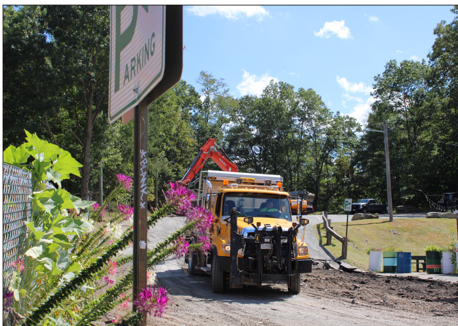
Sept. 3 — Pavement preparations at Narrowsburg, NY's municipal parking lot on Main Street.
