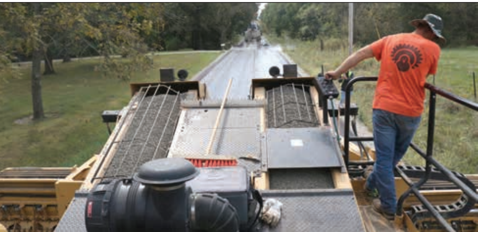
Pettis County Road Department worker Daniel Sparks stands on a top stone spreader as it lays a layer of rocks on Rattlesnake Road near Smithton in October 2021. In front, a truck lays down a layer of prime oil. This is part of the process of turning a gravel road into a chip and seal road.
