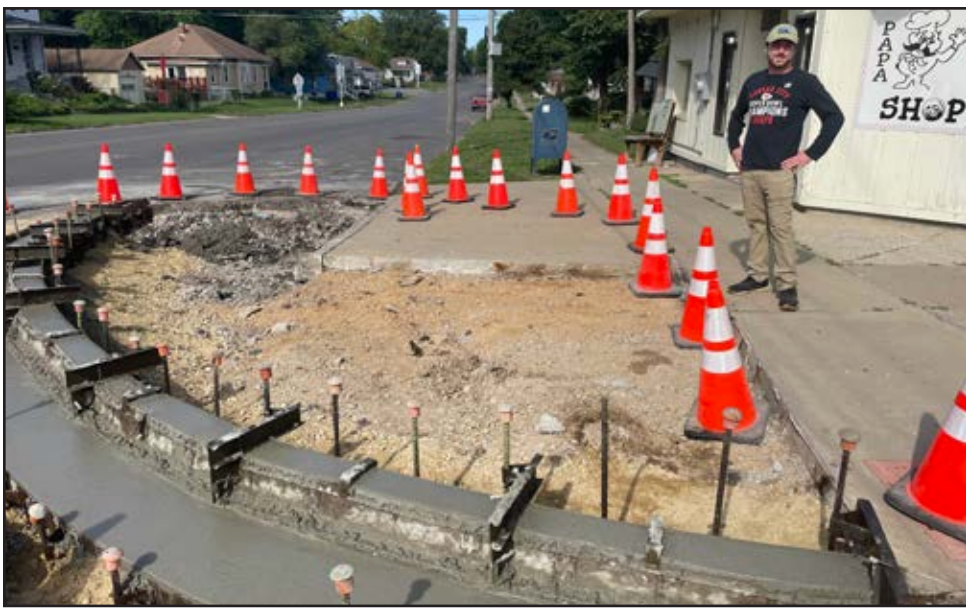
Ayden Bartley with Papa Jake's Donuts looks at the new bump-out in front of his shop. City planners hope the bump-outs and islands will give pedestrians refuge from West 16th Street traffic. PHOTO BY CHRIS HOWELL | DEMOCRAT
