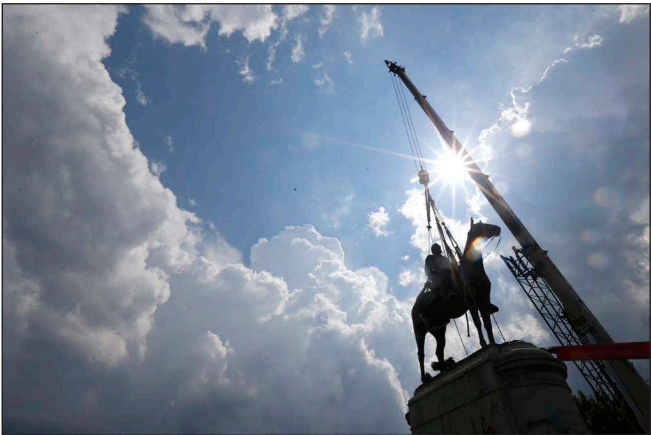
Work crews work to remove the statue of confederate general Stonewall Jackson, Wednesday, July 1, 2020, in Richmond, Va. Richmond, Virginia, has secured an $11 million philanthropic donation to build a new interpretive center city officials hope will someday be part of an ambitious, long-envisioned memorial campus honoring the memory of enslaved people. Richmond's grant is among more than $16 million in total funding The Mellon Foundation is providing to recipients in the former Confederate capital for projects that are “examining, preserving and reimagining” its “rich historical narratives:
