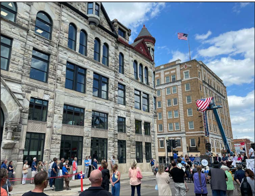
On Friday, May 5, the Historic Trust Building, 322 S. Ohio Ave., was reopened after a four-year restoration effort by CSC Construction Group. A crowd of well-wishers attended. PHOTO BY CHRIS HOWELL | DEMOCRAT
