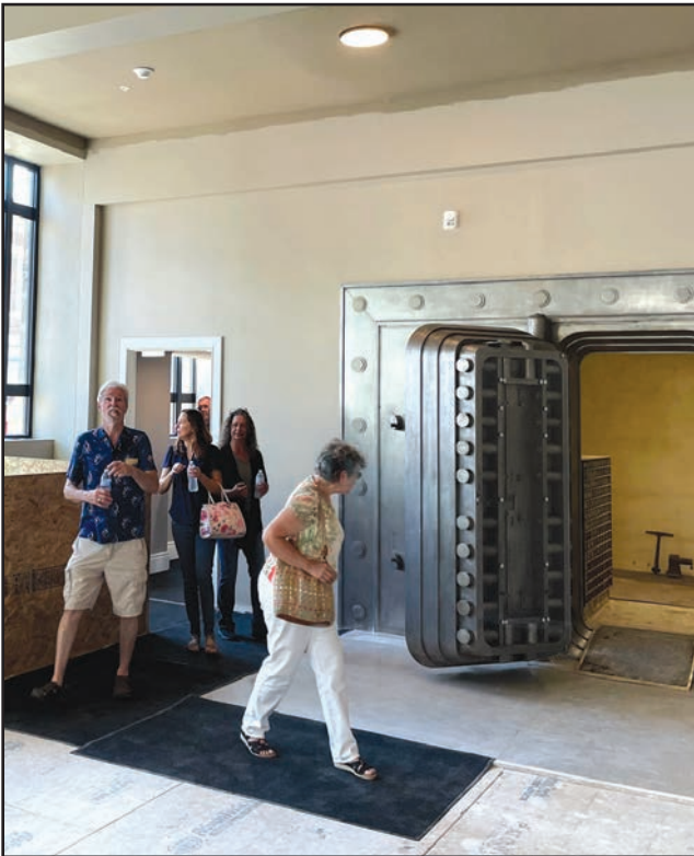
The ground floor will have marble floors and a room “safe” from any storm. Some items, like the safe and elevator shaft, had to be designed around rather than removed completely.
