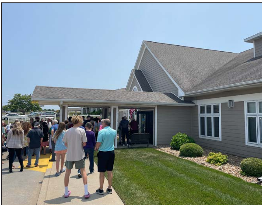
Primrose Retirement Community, 3751 W. 10th St. in Sedalia, houses 52 independent living apartment homes and 77 assisted living apartment homes with a maintenance free lifestyle.
