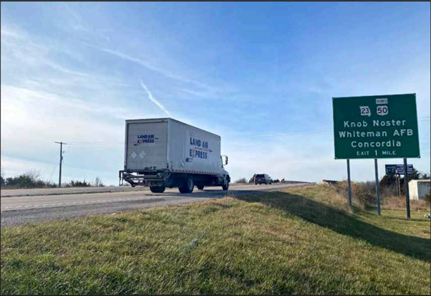
On Wednesday afternoon, Dec. 13, vehicles drive through Johnson County on Highway 50 as they approach the bridge over the Union Pacific Railroad in Knob Noster. MoDOT began rehabilitation work on the westbound bridge this week. FILE PHOTO BY NICOLE COOKE | WARRENSBURG STAR-JOURNAL
