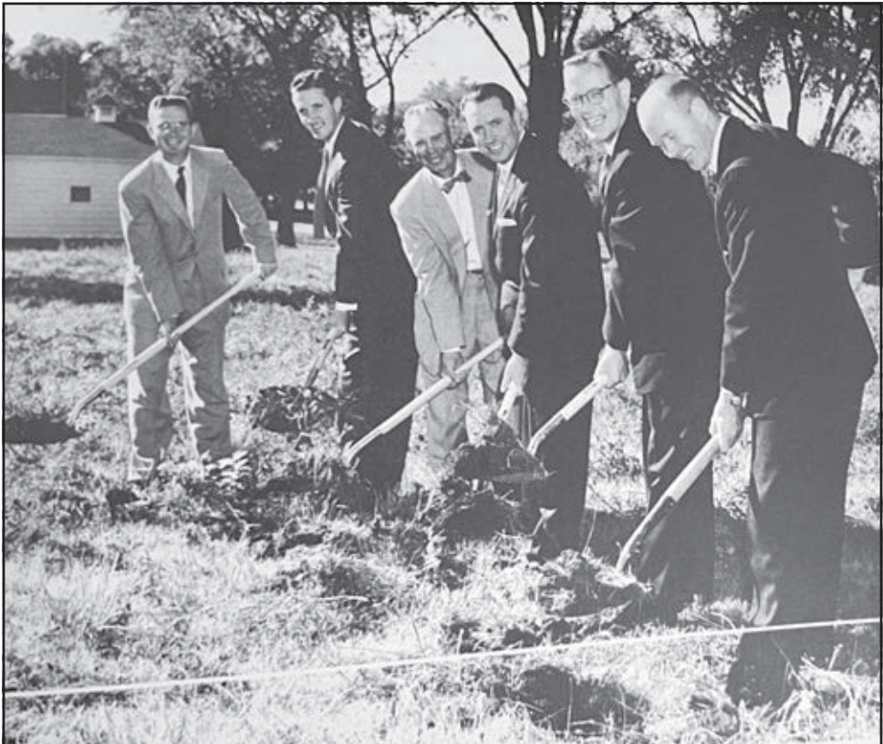
The groundbreaking for the new Sedalia LDS Chapel at South Park Avenue and West Broadway Boulevard occurred in the 1950s. The photo and article appeared in the Sedalia Democrat. The late Doyle Furnell was the project agent.
