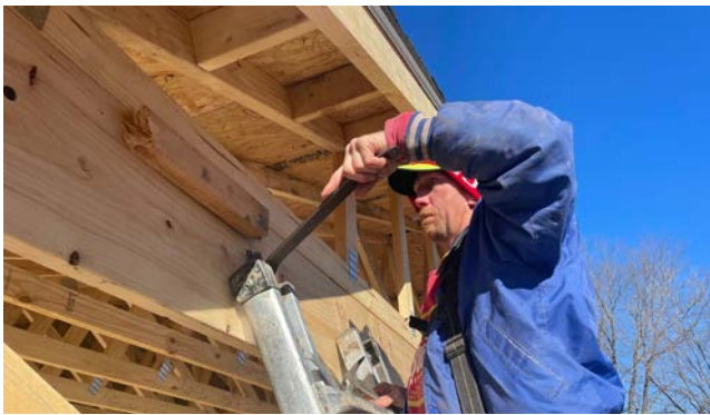
Tony Shepherd with Shep's Construction taught volunteers working on the 2023 Habitat for Humanity homes. This season one home is planned on East 25th Street at Lafayette Avenue. FILE PHOTO BY CHRIS HOWELL | DEMOCRAT
