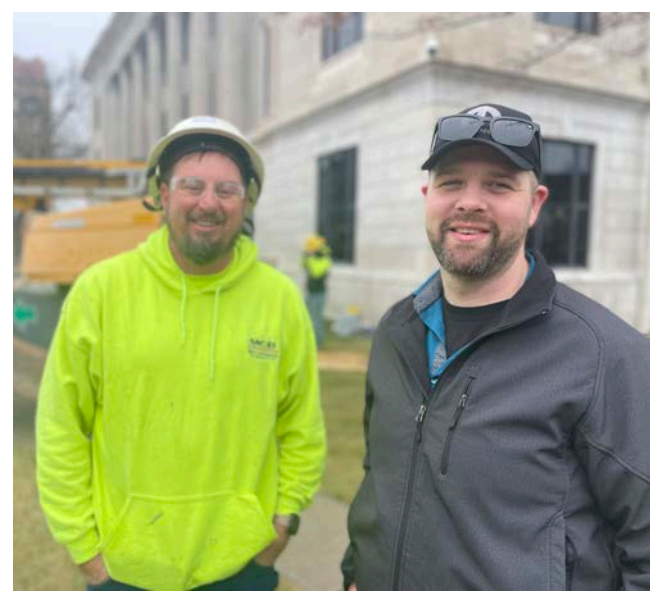
Superintendent Roy Bukowski with Mid-Continental Restoration out of Fort Scott, Kansas conducts a last day walk around the Pettis Courthouse with Pettis County Director of Buildings and Grounds Chris Hoke. Crews lay plywood ahead of their lift to avoid rutting the lawn.
