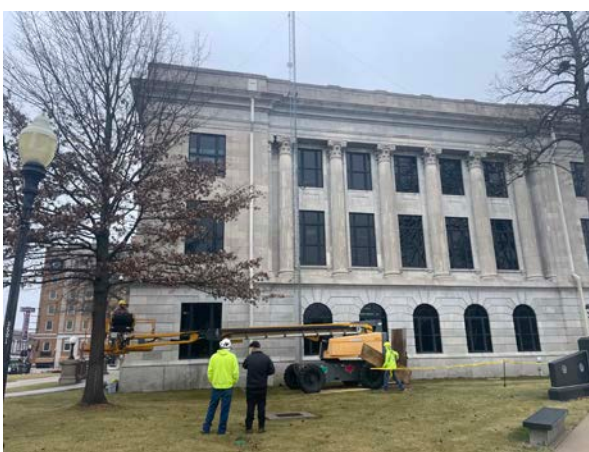
A masonry crew with Mid-Continental Restoration out of Fort Scott, Kansas wrapped up its restoration of the exterior of the Pettis County Courthouse on Thursday, Jan. 30. PHOTO BY CHRIS HOWELL | DEMOCRAT
