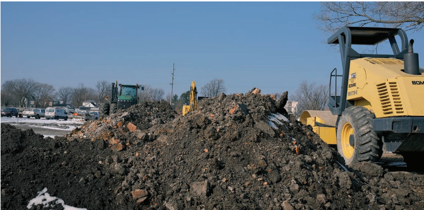
City officials said soil encountered (not pictured) on Friday, Jan. 16 was discovered by crews excavated for a stormwater retention basin near the Memory Lanes Bowling Alley and the new Fire Station on Sedalia’s east side. CHRIS HOWELL | DEMOCRAT
