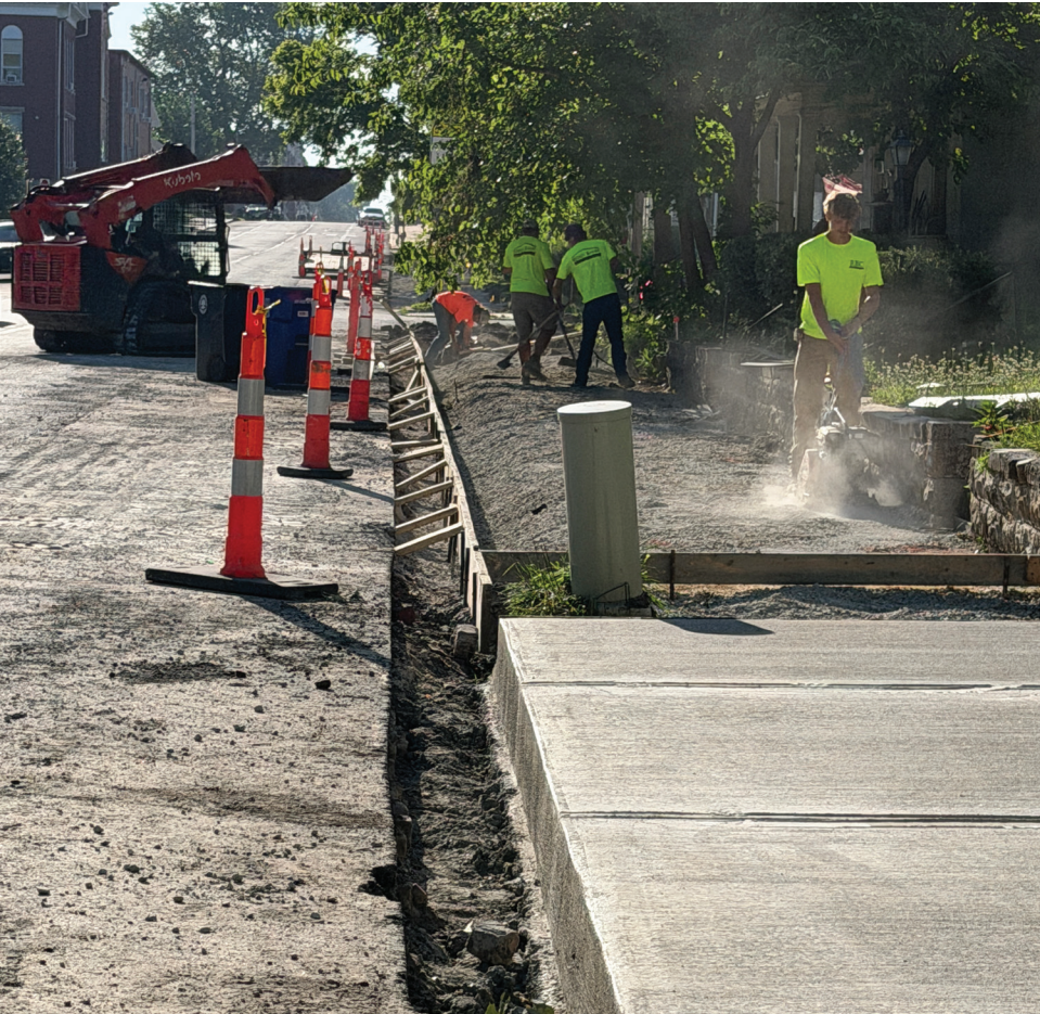
Crewmen with Rhad Baker Construction of Fulton are busy replacing the sidewalk along Third Street with a path wide enough to handle bikes and pedestrians from Liberty Park to the Katy Depot. PHOTO BY CHRIS HOWELL | DEMOCRAT
